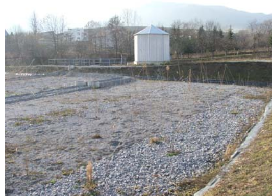
Krásna Lúka – 2007 (700 PE) Whole village connected with treatment plant Technology – 2x Imhoff tank, biofilter a 3 x 550 m2 wetlands. Village owns and takes care of WWTP – simple and low cost maintenance, system works with 2 pumps only
