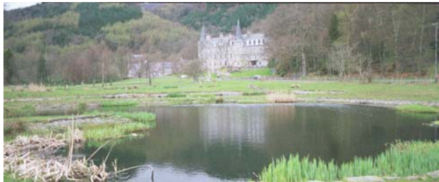
Hotel in Scotland with WSP (waste stabilisation pond)
