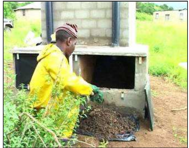
Fig.14: Emptying a UDDT faeces chamber (source: EWS.).
