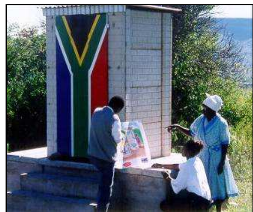
Fig. 3: A household with a UDDT is visited by a local facilitator (source: EWS).
