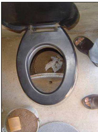
Fig. 12: Interior of a UDDT with sand container on the bottom left and plastic urine diversion pedestal from Atlas company at the top (source: EWS).
