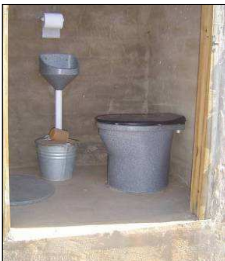
Fig. 11: Inside view of UDDT: urinal for men (left), bucket containing sand or ash, cover over second vault on the left side and urine diversion pedestal on the right (source: EWS).
