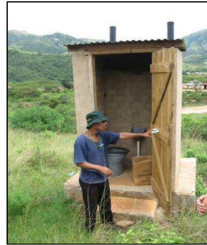
Fig. 5: Double vault UDDT in Maphephetheni in the eThekweni rural area (source: EWS).
