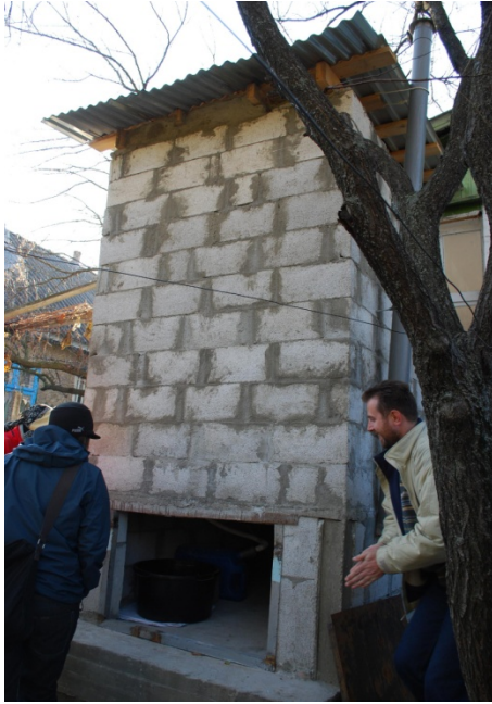
Figure 10 Ecosan toilet built with support from Wisdom (photo by Katja Larnholt).
