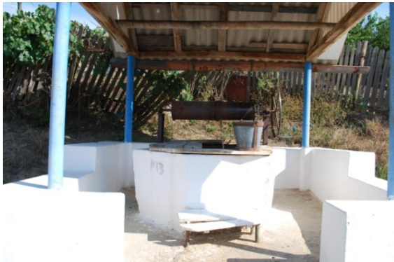
Figure 20 An improved dug well (including lid, roof and runoff protection).
