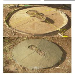
Fig. 6: Arborloo slab construction (source: ROSA Project, 2007)
