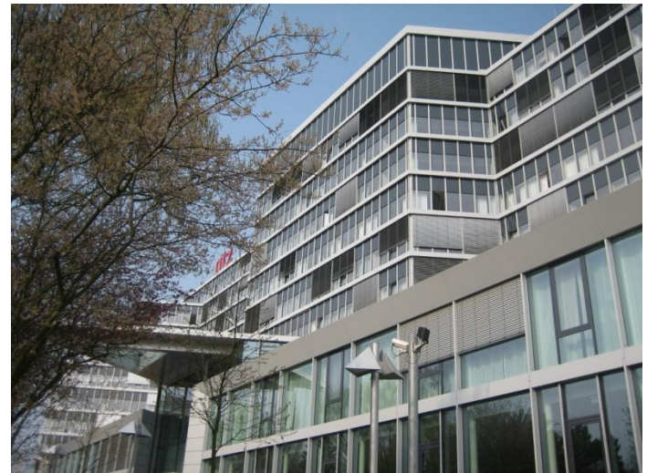
The renovated GTZ main building
