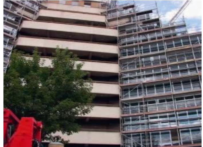
GTZ main office building during renovation
