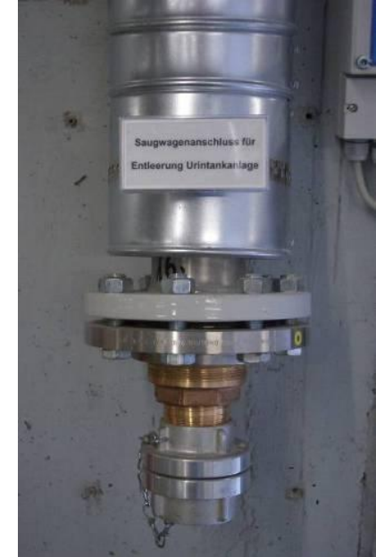
Docking station for vacuum tanker
