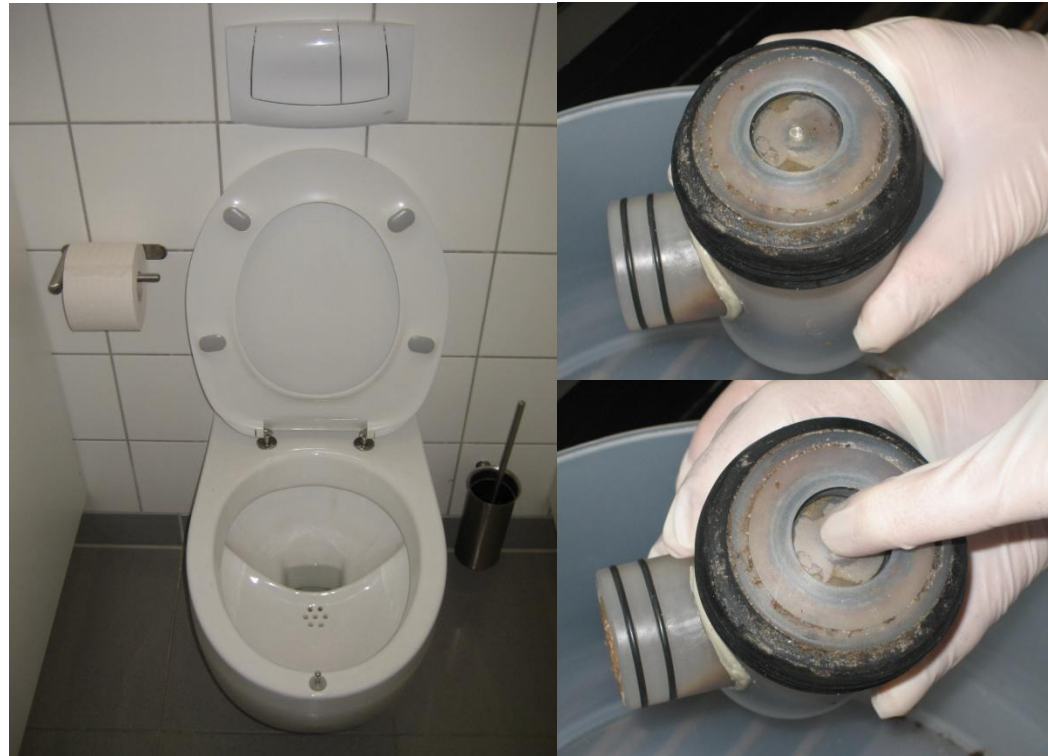
50 low-flush urine diversion toilets (Roediger) (1-3 L per urine flush, 6-9 L per faeces flush). Set during installation
