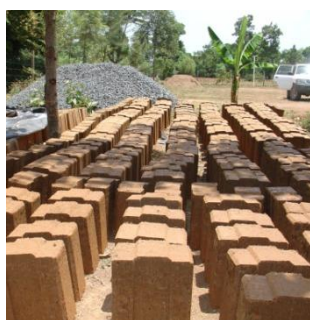
Fig. 9: Ready-made hydraform blocks
