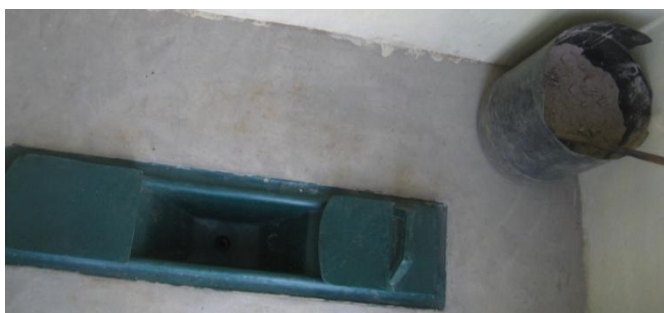
Fig. 4: Urine separating squatting pan and bucket with ash
