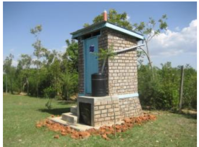
Fig. 3: Completed UDD toilet in Ugunja (source: GTZ EcoSan Kenya; photo taken in March 2009)
