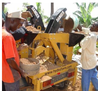
Fig. 8: Production of hydraform blocks
