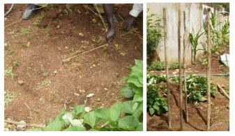
Fig. 4: Left: Marking out the circle. Right: Planting the poles. <u>Steps followed for the construction</u>
