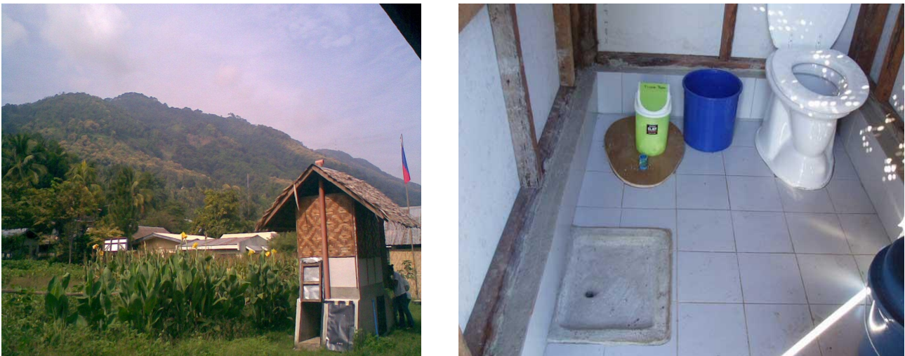
FIGURE 1 Double vault urine-diversion dehydration (UDD) toilet in one of the allotment gardens in Cagayan d'Oro. Left: outside view of toilet; right: inside view of toilet, with anal washing area at the front left (source: R. Holmer and http://puvep.xu.edu.ph/ecosan_toilet.htm )
