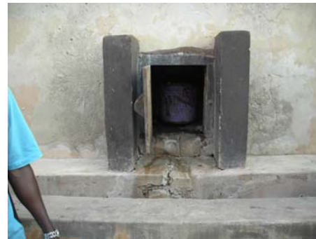
Figure 4 : Bucket latrines at Adoum sudurb.
