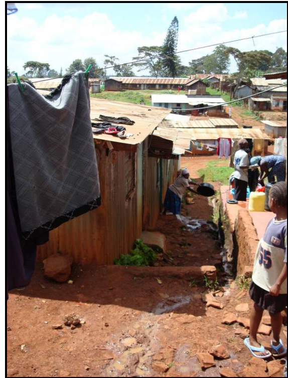
Figure 4-7: A woman discharging untreated greywater outside her house into an open drain
