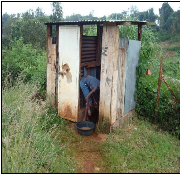
Figure 5-3: Greywater reuse at the household level for toilet cleaning (slab of a pit latrine) in Waruku
