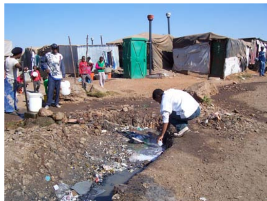
Figure D6.4: Stormwater drain at Freedom Square
