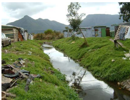
Figure D1.10: Stormwater channel to wetland, Masiphumelele
