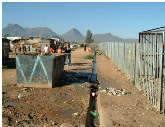
Figure D1.6: Stormwater channel at Fairyland
