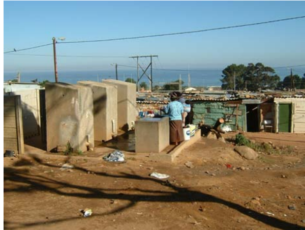
Figure D1.7: Communal toilets and washing facility at Kleinmond
