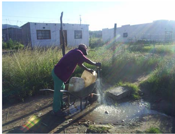
Figure D2.6: Flooded tapstand at Emahobeni
