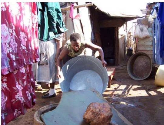
Figure D6.3: Greywater disposal down stormwater manhole
