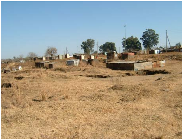
Figure D3.2: Shacks situated on moderate slopes on banks of Mzintlava River
