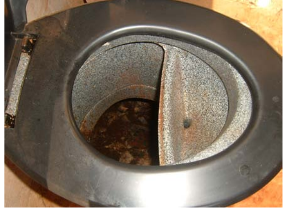
Figure D3.11: Mandela Park: Urine diversion toilets
