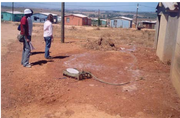
Figure D1.13: Water supply at Lingelethu
