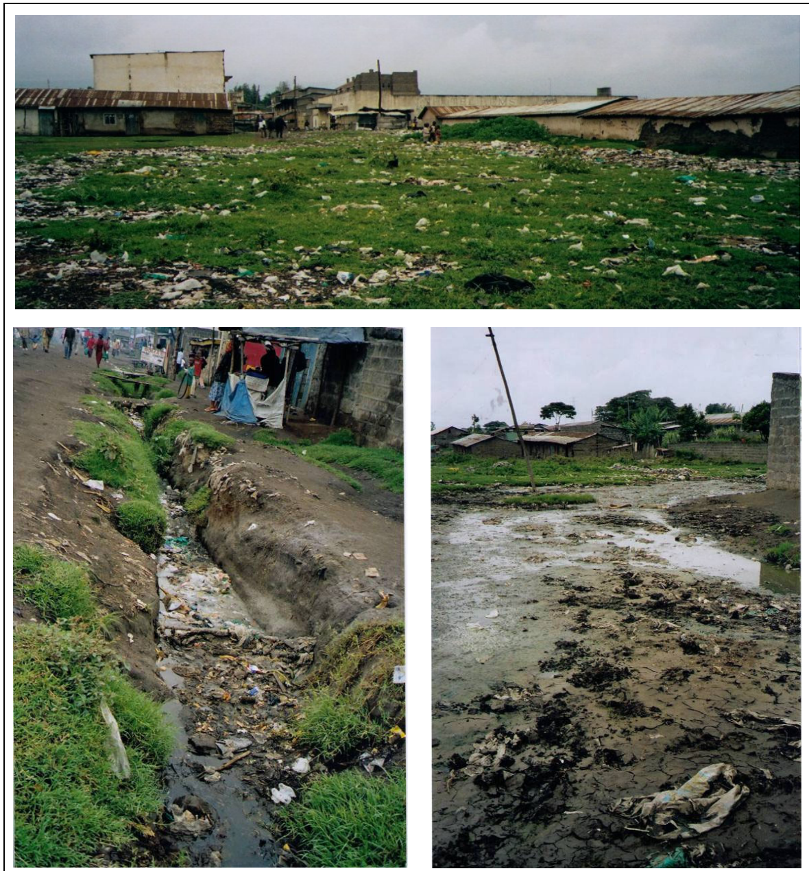
Figure 33: Top: Household waste polluting urban environment; Bottom left: Storm drainage filled with solid waste; Bottom right: Stormwater and greywater flooding a road;
