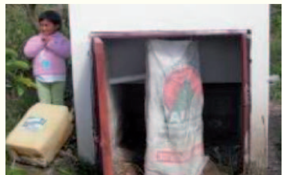
Figure 4: View of back door. Note the plastic bottle that collects urine and that the spaces around the door frame should be filled. (Photo: C. Canaday)
