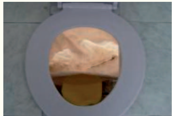
Figure 3: Seat, funnel and sack. The yellow plastic mesh keeps solids out of the funnel. Note that the rice sack, in this case, is too high. (Photo: C. Thibodeau)
