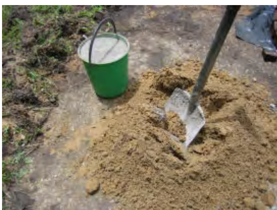
Make a mix of 10 litres cement and 50 litres clean river sand. Add about half of the mix to the brick mould and level off.
