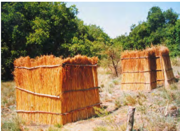
Left, the simplest superstructure – poles and grass – no door - no roof. Thanks to Jim Latham, Eco-Ed Trust. Right, more sophisticated pole and grass structure with door and roof. Durable door hinges can be made with cut sections of car tyres. Photo taken at Kufunda Village, Ruwa.
