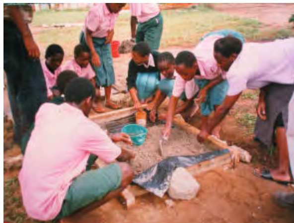
School children at the Mtomondoni Primary School learn how to make concrete slabs for eco-toilets
