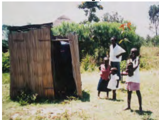
Left, simple portable structure made from poles and grass in Mozambique. This one has no door but has a roof, which has just been removed. The various sections are in panels and can be taken apart. Photo taken in Niassa Province. Thanks to Ned Breslin, WaterAid. Right, Arborloo structure built at Kusa Village, near Kisumu. Thanks to Osielana and RELMA
