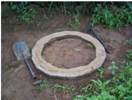
The ring beam has been embedded in levelled ground and the pit dug out to required depth. Soil extracted from the pit is placed around the ring beam. The slab is then fitted on the ring beam
