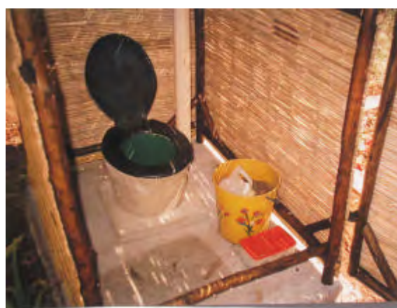
Fossa alterna at Woodhall Road, Harare. Note hand washing facility, waste water falling into a flower pot. Second pit during the first year was filled with leaves and compost. It was also used to grow comfrey (see later). Inside a home made pedestal has been fitted. The yellow bucket contains a mix of soil and wood ash and a dispenser. Leaves are also added occasionally.
