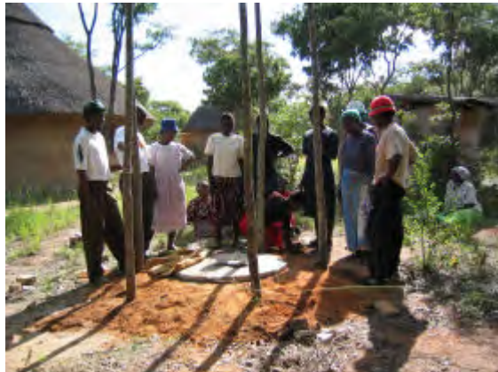
The slab is then moved and placed over the ring beam embedded in a layer of anthill mortar to keep it steady. The superstructure is now built with locally available materials like wooden poles and grass).
