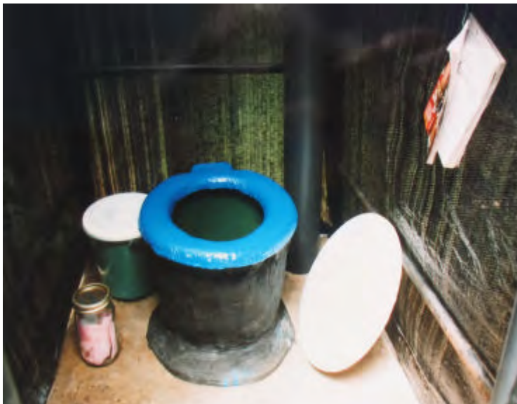
On the left the home made urine diversion unit is fitted over the slab. On the right the improved urine diverting pedestal, fitted with wooden seat. Note also the vent pipe fitted behind the pedestal to the right.
