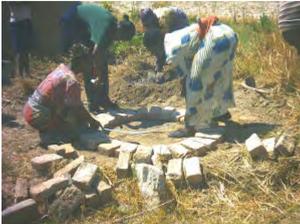
The ring beam is an important part of the structure, as it elevates the toilet slab above ground level and helps to protect the unlined shallow pit. Most ring beams are made with local fired bricks and termite mortar. The slab sits on top of the beam and then the structure is built around this. On the right a group of villagers attend the compost toilet workshop in Mondoro.
