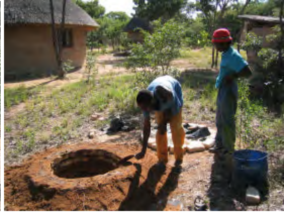
Digging pit inside brick ring beam
