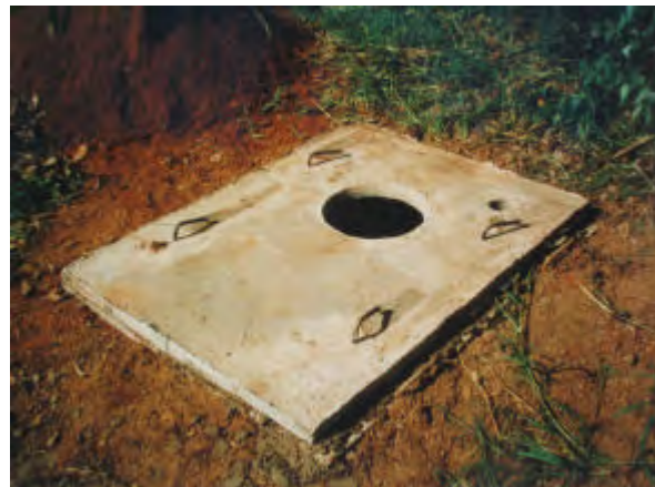
Adding a layer of weak cement mortar for the slab to rest on. This helps the slab to rest on the ring beam without strain. Also if a vent pipe is used, the pit should be air tight, thus allowing the suction of the pipe to draw air down the squat hole or pedestal. This leads to odourless conditions in the toilet. On the right a slab is mounted over the ring beam. This slab has a larger hole intended for a pedestal cast in it.
