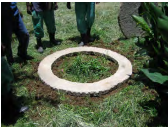
Digging pit inside concrete ring beam.
