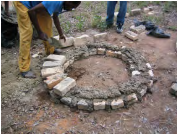
A brick ring beam being built at Kufunda training centre, Ruwa, Zimbabwe. In this case two courses of bricks are laid on top of each other without any corbelling as this is considered easier for villagers. The bricks are mortared with local ant hill soil which resists erosion. The 0.8m diameter hole is dug inside the ring beam and the soil placed around the ring beam and rammed in place. The 1m slab is then fitted.
