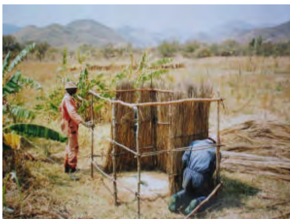
Simple Arborloo 's at the Eco-Ed Trust, Mutorashanga, Zimbabwe. The pole and grass structure is easily taken apart and reconstructed from the original materials. The grass can be replaced every year if required. This type does not have a roof, but a roof is desirable to keep out rain. Thanks to Jim Latham,
