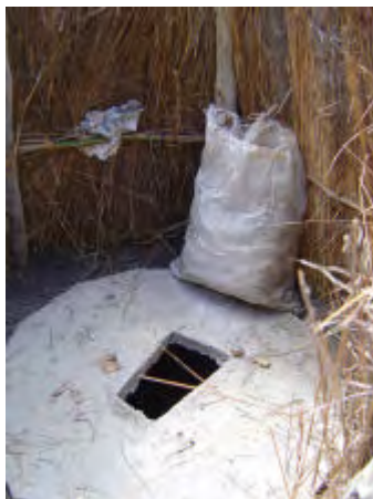
A sack of soil near the home made slab on an Arborloo . The finished Arborloo made in the simplest way, provides a safe way of disposing of excreta. The facility offers privacy, with almost no smell or fly nuisance. It is an important first step in the provision of sanitation for low income families. These photos were taken in the Mondoro district.
