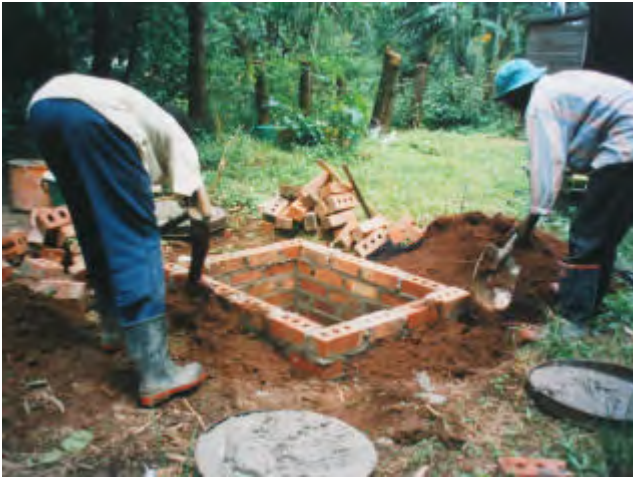
One of the two pits is dug and lined with cement mortared fired bricks. The steel frame (with door frame) is erected at the "door" end of the slab and the brick walls are built. "Sprags" of steel welded to the frame link the steel component with the brick and mortar work.
