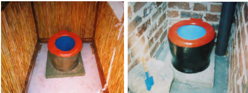
Home made pedestal placed on the slab. The pedestal is smart, cheap and durable.
