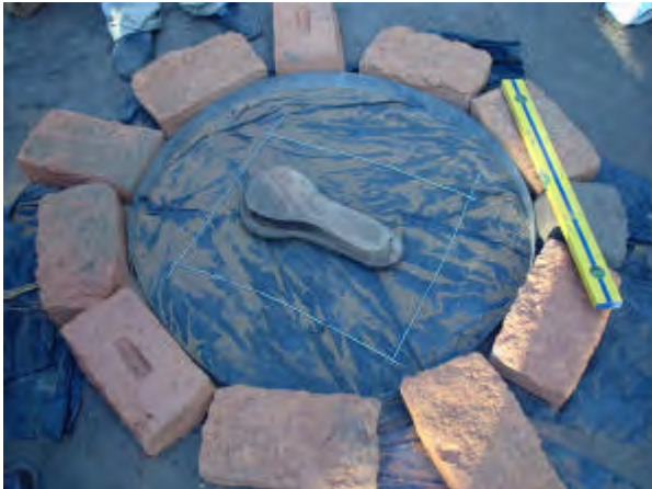
Making a round 0.8m diameter concrete slab in Malawi with sharp river sand and cement. When the river sand is of high quality, the addition of granite stones may be unnecessary. In this case a tin strip 40mm deep is formed into a circle 0.8m in diameter and supported by bricks. It is laid over a sheet of plastic. 4 wires are cut as reinforcing. In this case 2 metres of 2.5mm wire has been cut into 4 pieces (2 X 0.55m and 2 X 0.45m). 3mm or 4mm wire can also be used. The mix of sharp river sand and cement is 4 to 1 (20 litres river sand and 5 litres cement). 8 slabs can be made from one 50 kg bag of cement using this method. High quality river sand and proper curing are important.
