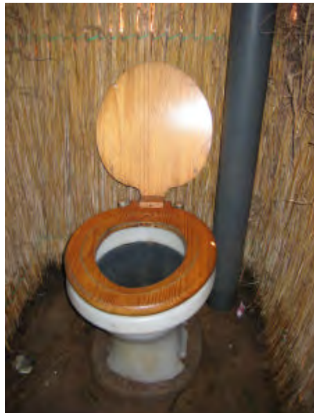
This Fossa alterna (using a 1.2m X 0.9m slab) has been upgraded first by adding a non urine diverting pedestal (left) and later by adding a urine diverting pedestal (right). When fitted to a shallow pit system the urine diverting pedestal is easier to install if the urine pipe lies above slab level.
