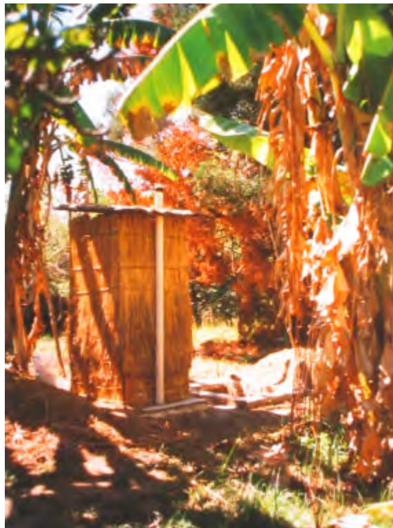
On the left the prototype Fossa alterna used a wooden structure and two shallow pits with brick ring beams. On the right a Fossa alterna in a low density suburb in Harare. This unit used two concrete ring beams, a structure made with a steel frame overlaid by grass and a 75mm PVC vent pipe.
