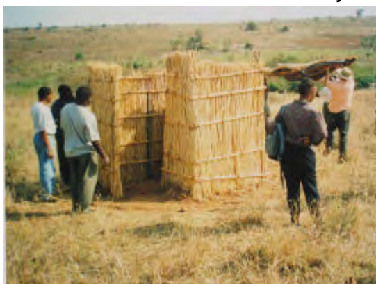
Left, simple portable structure made from poles and grass in Mozambique. This one has no door but has a roof, which has just been removed. The various sections are in panels and can be taken apart. Photo taken in Niassa Province. Thanks to Ned Breslin, WaterAid. Right, Arborloo structure built at Kusa Village, near Kisumu. Thanks to Osielana and RELMA
