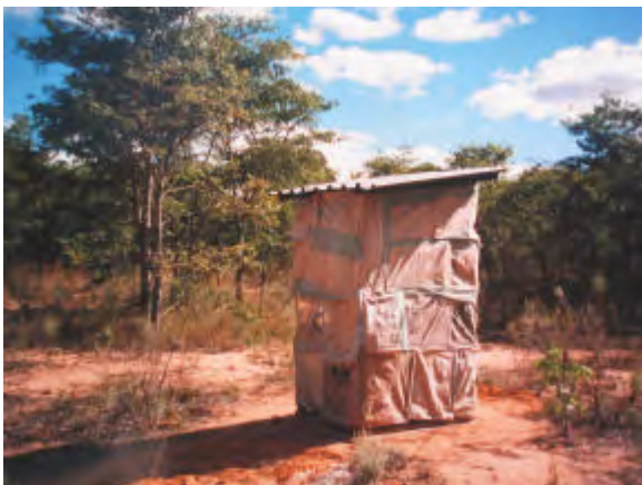
Structure using small gum poles and old cement packets – also with a door Photo taken at Kufunda Village Ruwa. Thanks to Marianne Knuth. Moving an Arborloo superstructure in Maputaland, South Africa. Note the wooden structure has legs. Thanks to Dave Still and Stephen Nash of Partners in Development.
