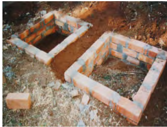
Prototype Fossa alterna being built at Woodhall Road. Each ring beam was constructed with three courses of cement mortared brickwork. The two pits were only 0.3m apart. This distance was later increased to 1m. The experimental prototype had a shallow pit only 0.6m deep. Later pits are dug over 1m deep, and normally at 1.2metres. 1.5 metres is a maximum depth for the Fossa alterna .
