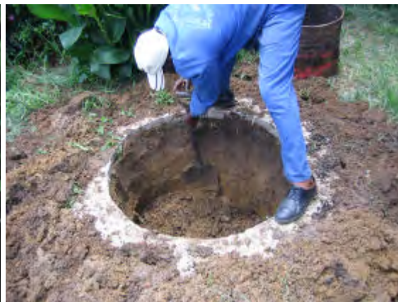
Digging pit inside concrete ring beam.
