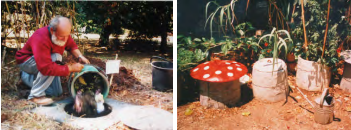
Tipping the contents of the bucket from a UD toilet into a small shallow pit for processing. The shallow pit is covered with a concrete lid with hole which is itself covered. On the left three cement jars are shown. The one actively being filled is covered with an attractive painted concrete cover.
