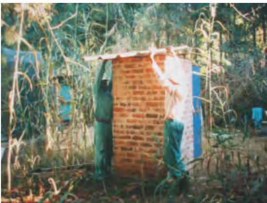
The roof is fitted after completion of the brickwork and door fitting. An asbestos pipe will also be fitted. Photo on right shows first stage of dismantling. The pipe, pedestal and roof have been removed. Now the brickwork is taken apart.
