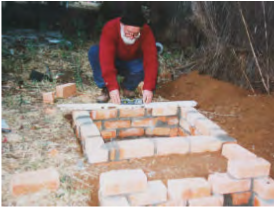
Prototype Fossa alterna being built at Woodhall Road. Each ring beam was constructed with three courses of cement mortared brickwork. The two pits were only 0.3m apart. This distance was later increased to 1m. The experimental prototype had a shallow pit only 0.6m deep. Later pits are dug over 1m deep, and normally at 1.2metres. 1.5 metres is a maximum depth for the Fossa alterna .
