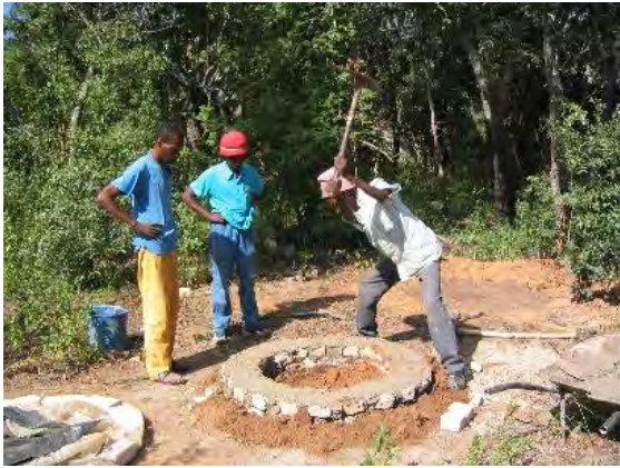
Digging pit inside brick ring beam
