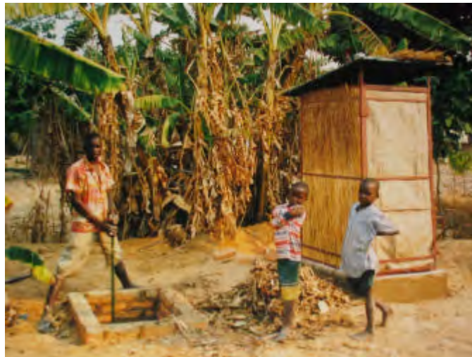
Fossa alterna in Epworth near Harare. It has two shallow pits, a single concrete slab and single superstructure, made with a light steel frame covered with grass. The Fossa alterna was initially designed for per-urban use on medium sized plots, but can be used on smaller plots and also in the rural areas.
