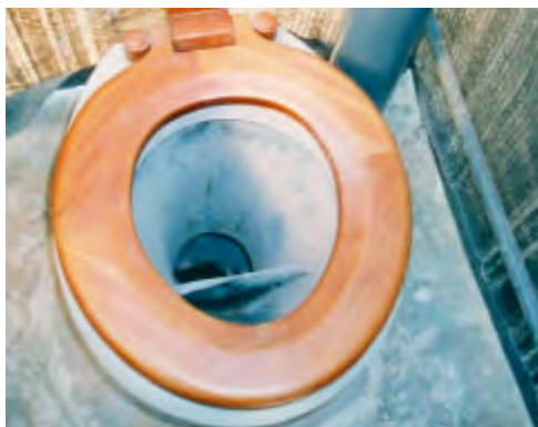
This urine diverting pedestal has been mounted on a 1.2m X 0.9m concrete slab mounted on an “above the ground” vault (see earlier chapter). In this case the urine pipe can be led off below slab level. The urine pipe is shown on the right leading to a plastic container. The two bricks which locate the bucket (not in place) which contains the faeces, soil and ash, are also shown.
