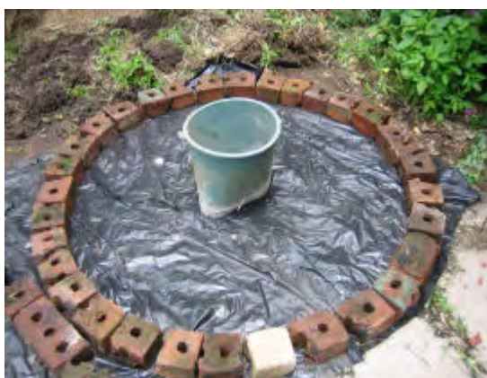
Lay a plastic sheet on level ground and lay bricks in circle 1.15m in diameter to make a mould. Add a shaped bucket or bricks to make the squat hole.
