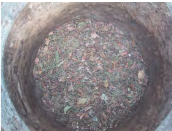
In a new series of experiments leaves are added to the bases of dug out pits and the users asked to put plenty of soil, ash and leaves into the pit as they use it. And not to use the pit as a garbage dump. It is thought that this refinement in the way pits are used will make hand excavation easy in the future. Where twin pits are used, the family alternates the use from one pit to the other. The pits under investigation are lined with concrete rings. Each concrete ring is 1m in diameter and 40cm deep. Up to 6 rings are used to line a pit. Pits of this size (1.8 cu.m.) can last a family up to 5 years.
