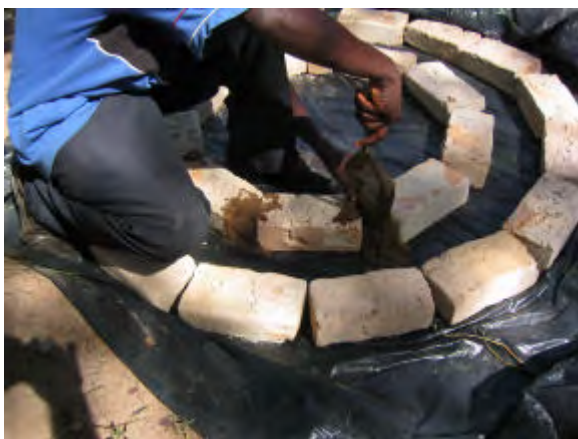
Two circles of bricks are laid over a plastic sheet. They are arranged so they form a mould in which the 6:1 mix of river sand (30 litres) and cement (5 litres) is placed. The open joints formed between the bricks of the inner circle of bricks can be filled with wet sand before adding the concrete mix. The mix is made in a wheel barrow and thoroughly mixed. Half the mix is added first to the mould. This is followed by a complete circle of 3 – 4mm wire. The remaining half of the mix is now added. The concrete is beaten down hard with bricks (see left photo) and smoothed down. The ring beam is then covered with plastic sheet and left over night. The following morning it is soaked in water and left to cure for 10 days. It is kept wet and under the plastic sheet throughout the curing period. After 10 days it can be lifted and placed on to the toilet site. A pit 1m – 1.5m is dug inside the ring beam. A sack of leaves is added and the concrete slab placed on top (in anthill mortar). The structure is then built around the slab. Soil, ash and leaves are added frequently to the pit contents to encourage the formation of good compost. For more detail see Appendix on low cost construction of Arborloo . Thanks to Marianne Knuth and Kufunda Village.
