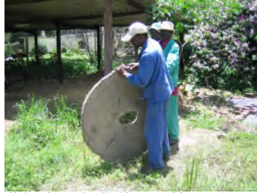
Round concrete ring beams and slabs can be made off the site and rolled into position as these photos show. In this case the larger ring beam (ID 1 metre) is being rolled onto site and fitted with a 1.15m diameter slab.
