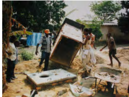
The 1.2mX 0.9m rectangular concrete slab has been used to build this Arborloo (left) and the Fossa alterna (right). Most Arborloo and Fossa alterna toilets use squat holes rather than pedestals. But they can be upgraded by adding pedestals and vent pipes. The vent pipe helps to remove smells and excess moisture from the pit
