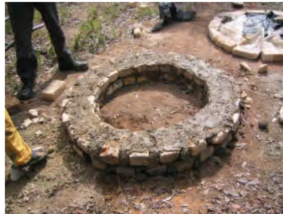
A brick ring beam being built at Kufunda training centre, Ruwa, Zimbabwe. In this case two courses of bricks are laid on top of each other without any corbelling as this is considered easier for villagers. The bricks are mortared with local ant hill soil which resists erosion. The 0.8m diameter hole is dug inside the ring beam and the soil placed around the ring beam and rammed in place. The 1m slab is then fitted.
