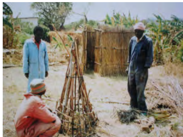
Simple Arborloo 's at the Eco-Ed Trust, Mutorashanga, Zimbabwe. The pole and grass structure is easily taken apart and reconstructed from the original materials. The grass can be replaced every year if required. This type does not have a roof, but a roof is desirable to keep out rain. Thanks to Jim Latham,
