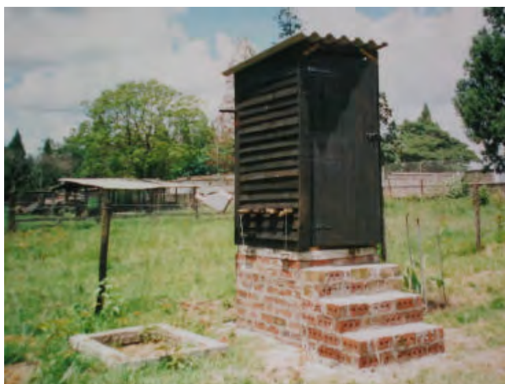
Vault above ground and pit below the ground – used alternately.
