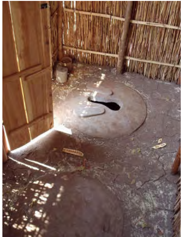
The interior of the structure shown above on right showing the two brick lined pits within the brick structure. On the left a demonstration structure showing one pit covered with a squatting slab and the other covered with a plain slab. Photo on left taken in Thyolo, photo on right taken in Phalome. Thanks to COMWASH
