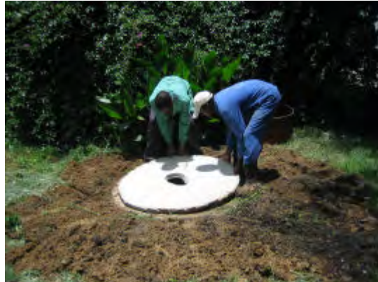
The ring beam has been embedded in levelled ground and the pit dug out to required depth. Soil extracted from the pit is placed around the ring beam. The slab is then fitted on the ring beam
