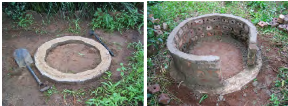
The 1 metre diameter concrete slab and matching ring beam can be made cheaply and is normally used to construct an Arborloo . But the same slab can be used on a Fossa alterna system (see earlier chapters). The same concrete slab and ring beam can be used to make a urine diverting toilet, as this sequence of photos shows. The ring beam has been laid down on level ground and backfilled with soil. A round brick wall is then built up on the ring beam to form a vault, with an opening at the rear, and high enough to accept a 20 litre bucket for containing the faeces, ash and soil.
