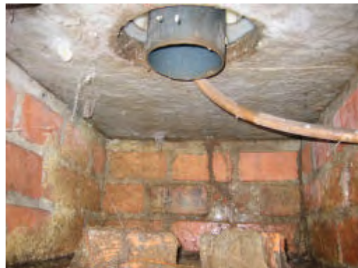
This urine diverting pedestal has been mounted on a 1.2m X 0.9m concrete slab mounted on an “above the ground” vault (see earlier chapter). In this case the urine pipe can be led off below slab level. The urine pipe is shown on the right leading to a plastic container. The two bricks which locate the bucket (not in place) which contains the faeces, soil and ash, are also shown.
