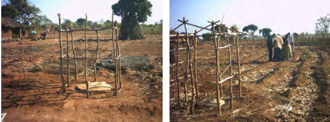
These Arborloos built in Embanweni, Malawi, where the soil is firm, do not have any form of pit protection. The 0.8m diameter concrete slab is laid directly over a 0.6m diameter hole and the simple superstructure built on top. The pits are dug about 1.0m deep.
