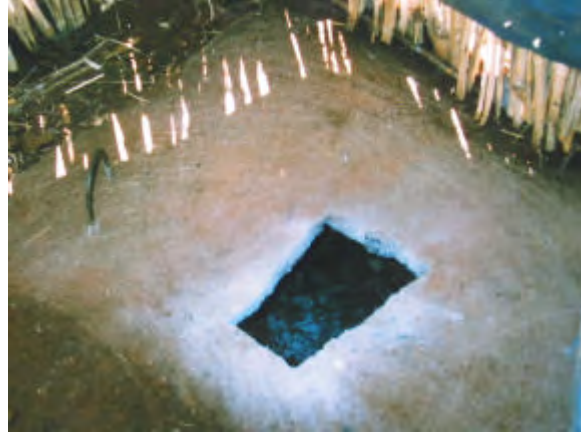
Arborloo structure with low cost vent pipe. On the left the structure is made of poles and grass with low cost vent made with sacking and cement slurry. The interior is shown on the right. Thanks to staff of Mvuramanzi Trust. Zimbabwe.
