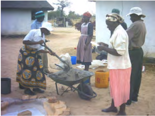
Participants at a “compost toilet workshop” in Mondoro are busy making the concrete slab. Instructions in the local language – Shona – are available. With the cement provided in the kit, a strong one metre diameter concrete slab can be built together with local river sand and some wire. The slab is flat and easy to construct. The importance of proper curing is emphasised. Cover with plastic sheet and after hardening keep wet for at least a week. The important aspect of this programme is that local villagers who are neither artisans or builders by trade acquire the skills. By far the greatest number of participants are women. In Mondoro, it is the women who train others to make the slab and toilet.
