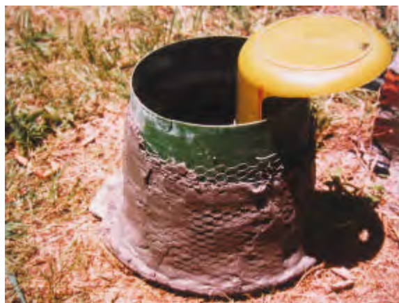
Stages in making one "home made version" of a urine diverting pedestal. Urine in this case ran down through the hole into another plastic bucket held within the vault and then to a soakaway.
