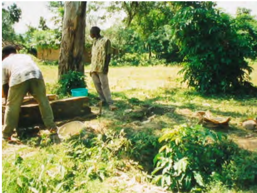
A new latrine is being built to the left. On the right is the depression left from an old latrine pit. Close inspection reveals that an indigenous tree is starting to grow there. Photo a Kusa Village, Kenya.
