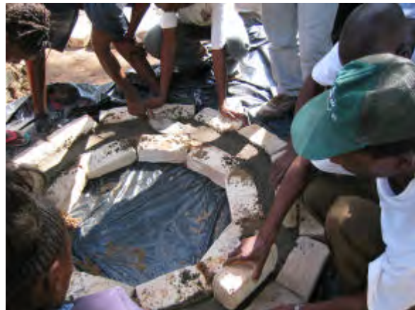
Two circles of bricks are laid over a plastic sheet. They are arranged so they form a mould in which the 6:1 mix of river sand (30 litres) and cement (5 litres) is placed. The open joints formed between the bricks of the inner circle of bricks can be filled with wet sand before adding the concrete mix. The mix is made in a wheel barrow and thoroughly mixed. Half the mix is added first to the mould. This is followed by a complete circle of 3 – 4mm wire. The remaining half of the mix is now added. The concrete is beaten down hard with bricks (see left photo) and smoothed down. The ring beam is then covered with plastic sheet and left over night. The following morning it is soaked in water and left to cure for 10 days. It is kept wet and under the plastic sheet throughout the curing period. After 10 days it can be lifted and placed on to the toilet site. A pit 1m – 1.5m is dug inside the ring beam. A sack of leaves is added and the concrete slab placed on top (in anthill mortar). The structure is then built around the slab. Soil, ash and leaves are added frequently to the pit contents to encourage the formation of good compost. For more detail see Appendix on low cost construction of Arborloo . Thanks to Marianne Knuth and Kufunda Village.
