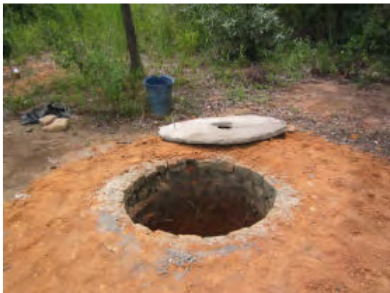
The slab is then moved and placed over the ring beam embedded in a layer of anthill mortar to keep it steady. The superstructure is now built with locally available materials like wooden poles and grass).
