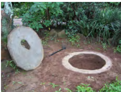
The same sequence using the smaller 0.85m internal diameter ring beam and one metre diameter slab. The hole is dug inside the ring beam down to a depth of 1 to 1.5 metres. The excavated soil is placed around the ring beam and rammed in place. The slab is then embedded on a layer of clay, weak cement or termite mortar laid on the ring beam, Now the superstructure must be built around the slab.
