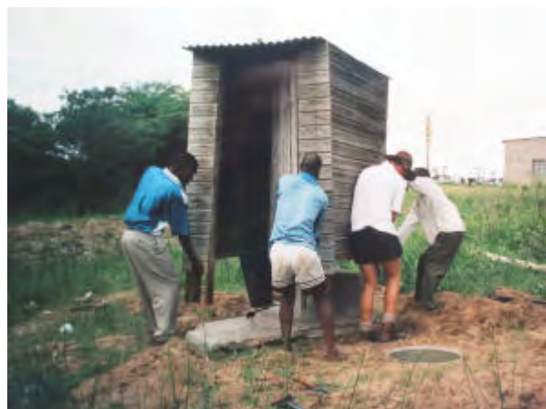
Structure using small gum poles and old cement packets – also with a door Photo taken at Kufunda Village Ruwa. Thanks to Marianne Knuth. Moving an Arborloo superstructure in Maputaland, South Africa. Note the wooden structure has legs. Thanks to Dave Still and Stephen Nash of Partners in Development.
