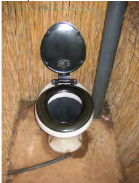
This Fossa alterna (using a 1.2m X 0.9m slab) has been upgraded first by adding a non urine diverting pedestal (left) and later by adding a urine diverting pedestal (right). When fitted to a shallow pit system the urine diverting pedestal is easier to install if the urine pipe lies above slab level.
