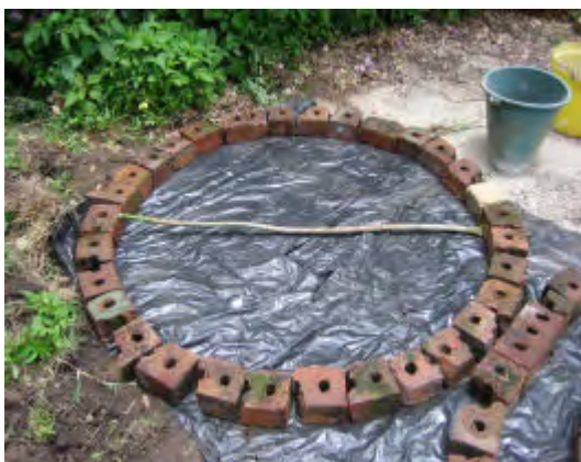
Lay a plastic sheet on level ground and lay bricks in circle 1.15m in diameter to make a mould. Add a shaped bucket or bricks to make the squat hole.
