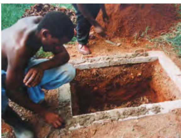
Adding a layer of weak cement mortar for the slab to rest on. This helps the slab to rest on the ring beam without strain. Also if a vent pipe is used, the pit should be air tight, thus allowing the suction of the pipe to draw air down the squat hole or pedestal. This leads to odourless conditions in the toilet. On the right a slab is mounted over the ring beam. This slab has a larger hole intended for a pedestal cast in it.
