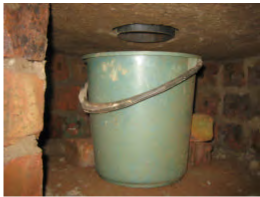
The one metre diameter slab has been fitted and bonded on top of the round vault in cement mortar and a urine diverting pedestal fitted. This could also be a squatting type urine diverting platform. The bucket is located in position under the urine diverting pedestal with some bricks.
