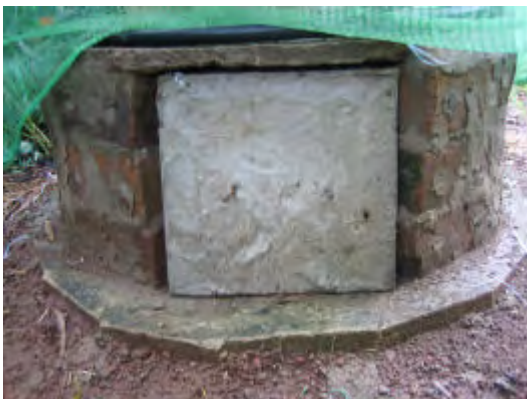
A concrete vault access door has also been made and fitted to the rear of the vault
