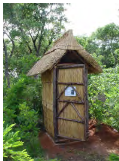
Left, the simplest superstructure – poles and grass – no door - no roof. Thanks to Jim Latham, Eco-Ed Trust. Right, more sophisticated pole and grass structure with door and roof. Durable door hinges can be made with cut sections of car tyres. Photo taken at Kufunda Village, Ruwa.
