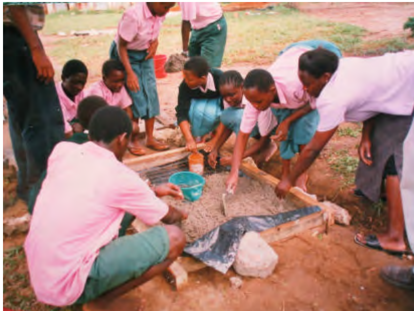
Concrete slabs are a very important part of the structure of all pit toilets. They are not difficult to make if the simple constructional details are followed. Making concrete components is a very good way of investing money for the future. If well made, concrete lasts almost for ever. Here school children make a concrete slab in Mombasa, Kenya
