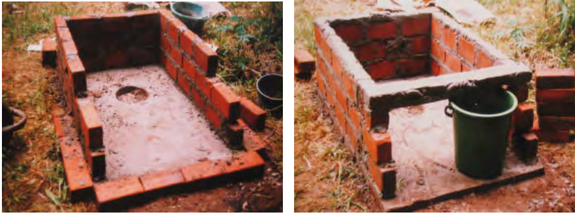
Stages in making the vault. The brickwork
