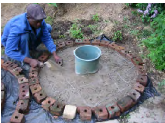
Add lengths of 3mm wire across the slab as reinforcing. At least four 1 metre lengths of wire are required, 2 in each direction. Add more wire if it is available. Then add the remainder of the concrete mix and level off. The squat hole mould can be removed with care once the slab has started to harden. The slab must now be cured. This means allowing it to harden overnight, then covering and watering down. The slab must be kept wet for at least 7 days to cure. 10 days is better. It must not be allowed to dry out. When thoroughly cured and strengthened it can be moved to the toilet site. The ring beam is laid down first on levelled ground, the pit dug and the slab added.
