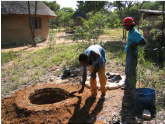
The pit is dug out down to 1 – 1.5 metres and the extracted soil placed around the ring beam and rammed in place. The ring beam and surrounding soil will help to make the toilet stable.
