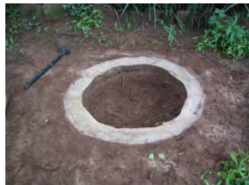
The ring beam has been embedded in levelled ground and the pit dug out to required depth. Soil extracted from the pit is placed around the ring beam. The slab is then fitted on the ring beam
