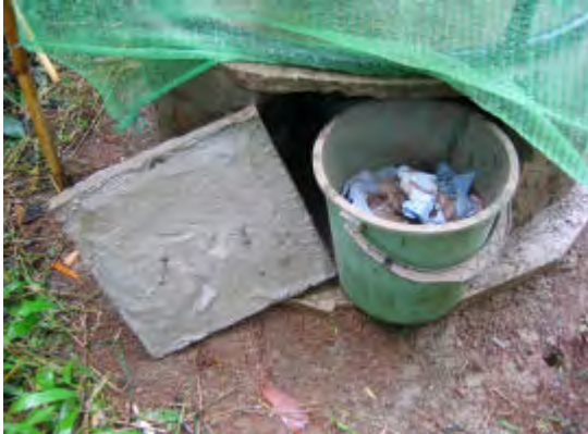
A concrete vault access door has also been made and fitted to the rear of the vault
