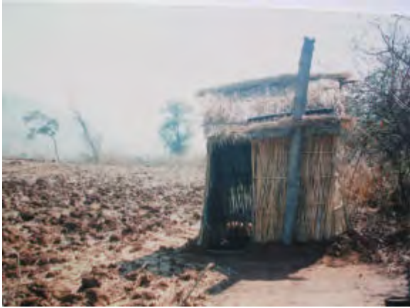
Arborloo structure with low cost vent pipe. On the left the structure is made of poles and grass with low cost vent made with sacking and cement slurry. The interior is shown on the right. Thanks to staff of Mvuramanzi Trust. Zimbabwe.
