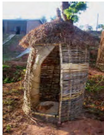
Woven basket superstructure from Malawi. Thanks to Steven Sugden and WaterAid. Woven basket structure on Arborloo in Northern Malawi. The door is made from sacking. A neat and effective unit. Photo: thanks to Jim McGill, Embangweni eco-san project.
