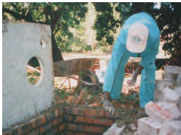
All the brickwork has been taken apart. The bricks are cleaned up. This is easy because the mortar is weak (20:1 sand and cement). On the right the same slab, having been removed from the original pit, is relocated on the second pit and mounted over a bed of weak cement mortar.
