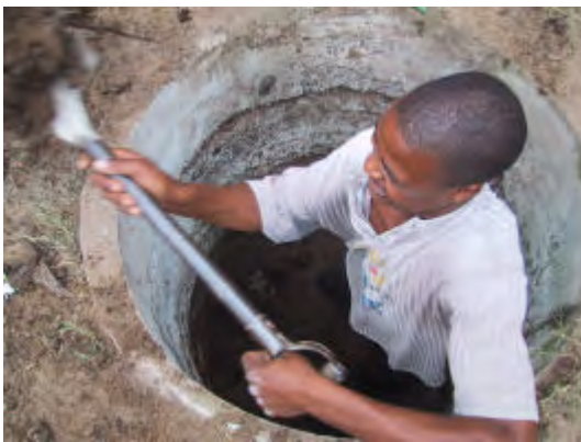
Some work on recycling the existing pit contents of VIP toilets is also being carried out in Maputaland. On the left a previously full pit toilet, to which soil and leaves were added from the top is being dug out three years later. Previously it would have been impossible to dig out by hand. In Maputaland and elsewhere in South Africa, large numbers of VIP toilets were built years ago and many are now full.
