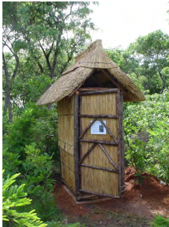
Compost toilet built above a shallow pit
