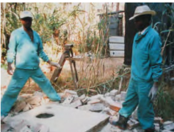
All the brickwork has been taken apart. The bricks are cleaned up. This is easy because the mortar is weak (20:1 sand and cement). On the right the same slab, having been removed from the original pit, is relocated on the second pit and mounted over a bed of weak cement mortar.
