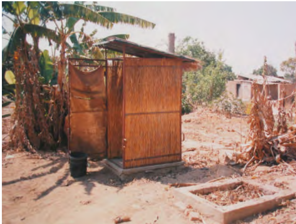
A Fossa alterna in Epworth, Zimbabwe. The twin pit system makes humus
