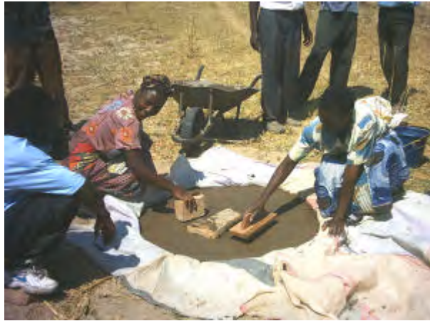
Participants at a “compost toilet workshop” in Mondoro are busy making the concrete slab. Instructions in the local language – Shona – are available. With the cement provided in the kit, a strong one metre diameter concrete slab can be built together with local river sand and some wire. The slab is flat and easy to construct. The importance of proper curing is emphasised. Cover with plastic sheet and after hardening keep wet for at least a week. The important aspect of this programme is that local villagers who are neither artisans or builders by trade acquire the skills. By far the greatest number of participants are women. In Mondoro, it is the women who train others to make the slab and toilet.
