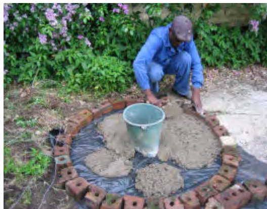
Make a mix of 10 litres cement and 50 litres clean river sand. Add about half of the mix to the brick mould and level off.
