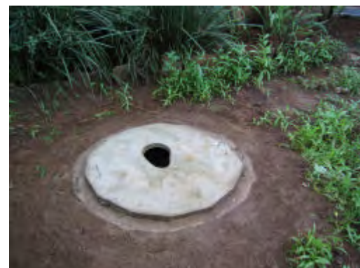
The same sequence using the smaller 0.85m internal diameter ring beam and one metre diameter slab. The hole is dug inside the ring beam down to a depth of 1 to 1.5 metres. The excavated soil is placed around the ring beam and rammed in place. The slab is then embedded on a layer of clay, weak cement or termite mortar laid on the ring beam, Now the superstructure must be built around the slab.
