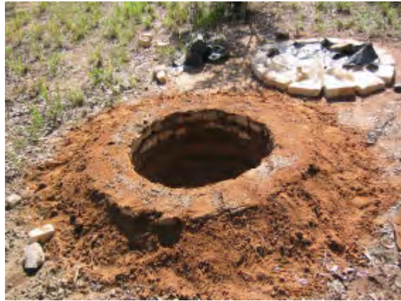
The pit is dug out down to 1 – 1.5 metres and the extracted soil placed around the ring beam and rammed in place. The ring beam and surrounding soil will help to make the toilet stable.
