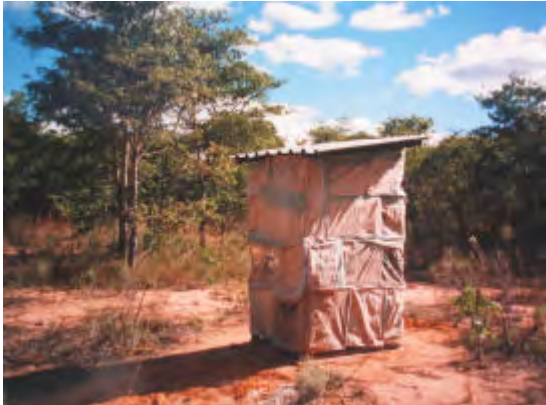
The 1.2mX 0.9m rectangular concrete slab has been used to build this Arborloo (left) and the Fossa alterna (right). Most Arborloo and Fossa alterna toilets use squat holes rather than pedestals. But they can be upgraded by adding pedestals and vent pipes. The vent pipe helps to remove smells and excess moisture from the pit
