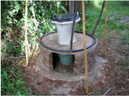
The one metre diameter slab has been fitted and bonded on top of the round vault in cement mortar and a urine diverting pedestal fitted. This could also be a squatting type urine diverting platform. The bucket is located in position under the urine diverting pedestal with some bricks.
