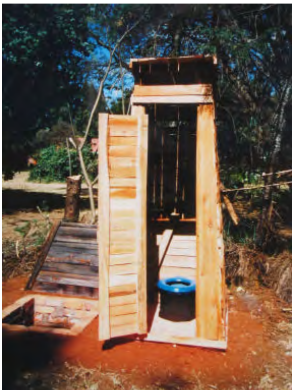
On the left the prototype Fossa alterna used a wooden structure and two shallow pits with brick ring beams. On the right a Fossa alterna in a low density suburb in Harare. This unit used two concrete ring beams, a structure made with a steel frame overlaid by grass and a 75mm PVC vent pipe.
