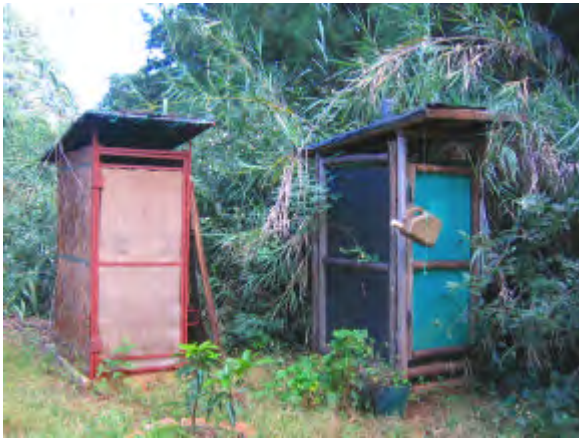
Two portable structures at Woodhall Road, Harare. One made of gum poles in sections which are wired together (right). The structure on the left is a steel frame covered with grass walling. Note hand washing device hanging from structure. All toilets should be provided with a hand washing facility. The structure made with steel frame and grass covering is easy to move. This is an excellent system where the frame is light and very durable and will last for many years. Less durable low cost walling materials like grass can be replaced when required. Photo taken at Fambidzanai, near Harare.
