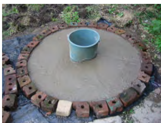
Add lengths of 3mm wire across the slab as reinforcing. At least four 1 metre lengths of wire are required, 2 in each direction. Add more wire if it is available. Then add the remainder of the concrete mix and level off. The squat hole mould can be removed with care once the slab has started to harden. The slab must now be cured. This means allowing it to harden overnight, then covering and watering down. The slab must be kept wet for at least 7 days to cure. 10 days is better. It must not be allowed to dry out. When thoroughly cured and strengthened it can be moved to the toilet site. The ring beam is laid down first on levelled ground, the pit dug and the slab added.
