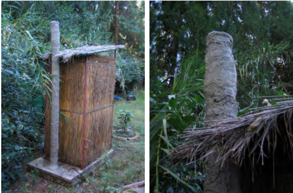
A durable home made vent pipe constructed from Hessian and a sand cement slurry with some wire reinforcing. Very effective and longlasting.
