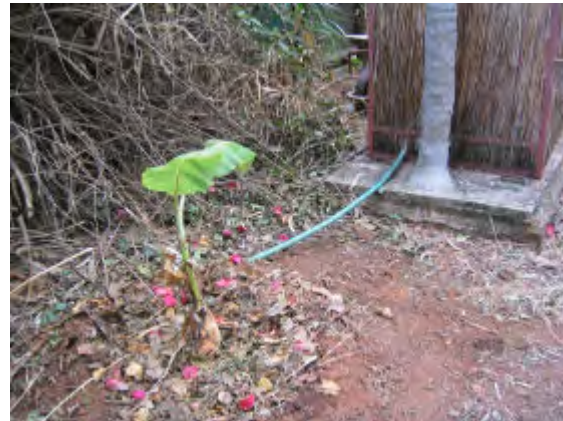
The urine diverting pedestal can be fitted into a single or double vault dehydrating or composting toilet. It can also be fitted over a shallow pit toilet. The urine pipe can be led into a soakaway or into a vegetable garden, preferably beneath ground level. It can also be led to a tree like a banana, as shown above. The urine can also be led to a plastic container placed in a hole dug in the ground. It is advisable to protect the pipe in some way by covering with soil etc. Here the pipe is exposed for the photo.
