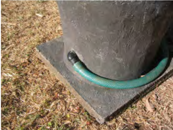
The urine outlet pipe has been added to the polyethylene pipe bend. This is led back over the concrete base of the urine diverting pedestal to the rear of the toilet.
