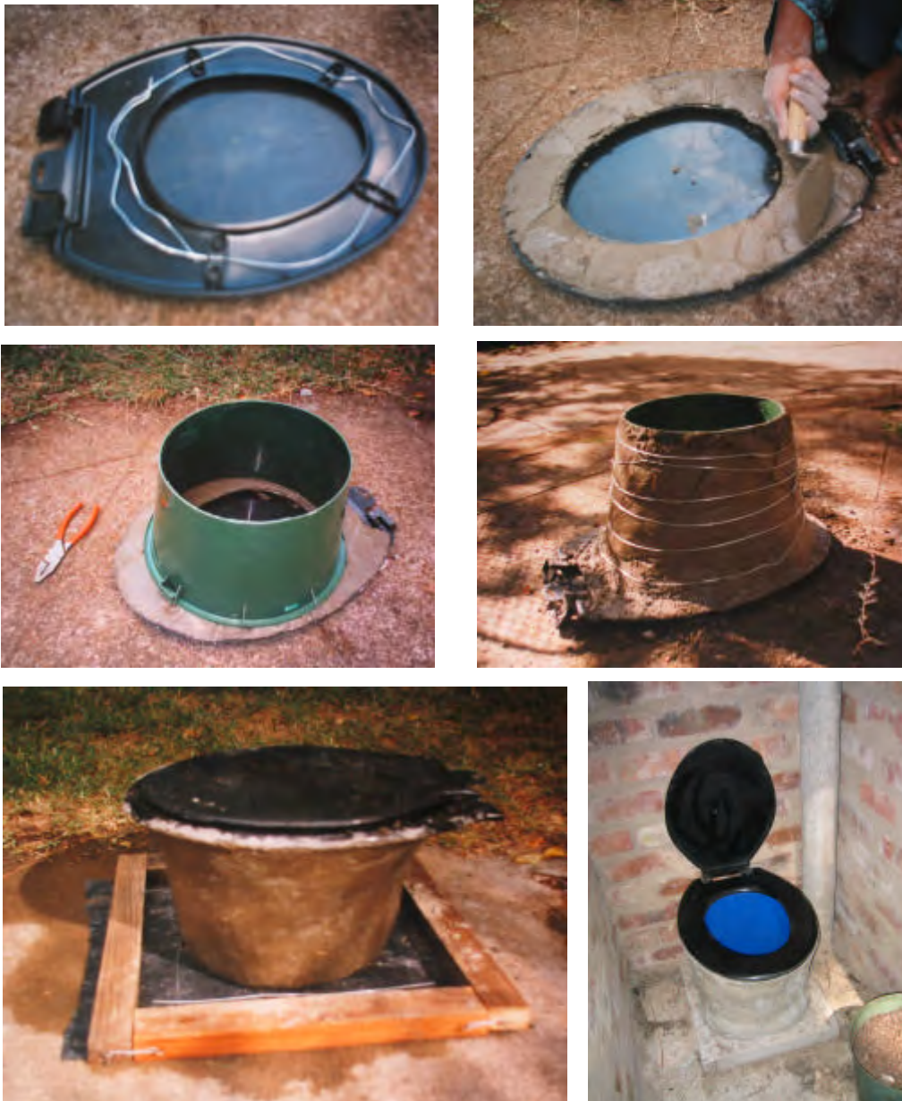
Finally a strong durable pedestal is made
