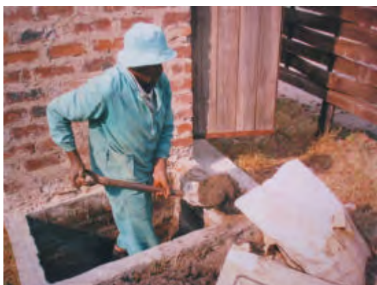
Compost being excavated from a Fossa alterna pit at the Friend Foundation, Harare (left) and in Niassa Province, Mozambique (right), a project of WaterAid. It is best placed in bags for storage first, and then mixed with topsoil and applied to vegetable gardens or containers. It can also be mixed with topsoil.
