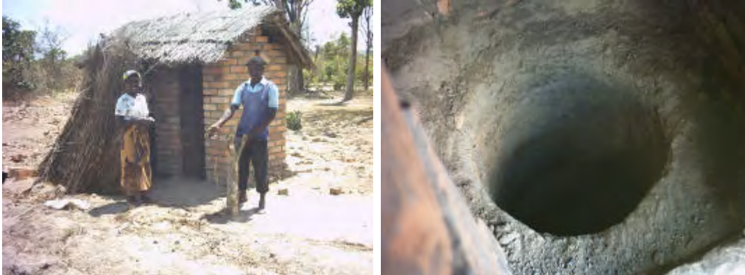
The Fossa alterna of Mr and Mrs Nyirenda of Yazoza Village, Embangweni, Malawi. The soil is hard and there was no need for a pit lining. The humus had recently been dug out of the pit (right).
