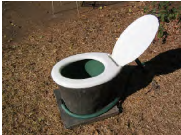
The urine outlet pipe has been added to the polyethylene pipe bend. This is led back over the concrete base of the urine diverting pedestal to the rear of the toilet.
