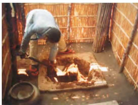
Compost being excavated from a Fossa alterna pit at the Friend Foundation, Harare (left) and in Niassa Province, Mozambique (right), a project of WaterAid. It is best placed in bags for storage first, and then mixed with topsoil and applied to vegetable gardens or containers. It can also be mixed with topsoil.
