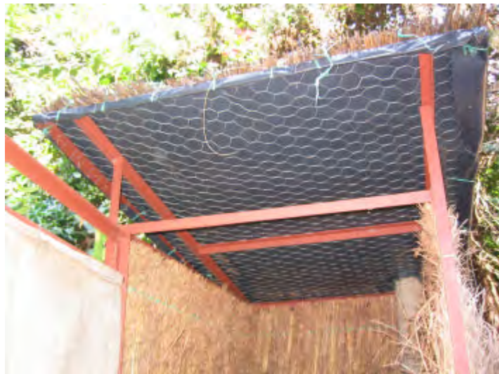
Close up of upper parts of the frame and roof
