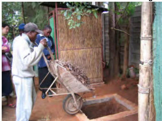
Next a thick layer of leaves is added to the base of the new pit. A layer of very weak cement mortar is added to the ring beam and the slab (in this case fitted with a plush pedestal) is lowered on to the ring beam. Finally the structure is fitted back over the slab. Good for another year.
