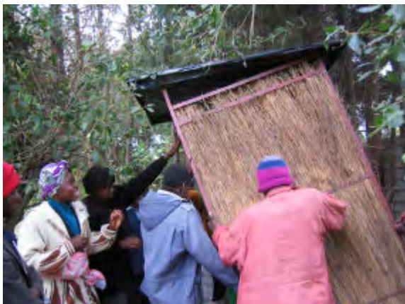
First, the structure and slab are removed from the pit which has been in use for one year. The pit contents are then covered with a good later of soil and leaves (right).
