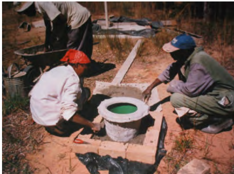
Making a low cost pedestal at Kafunda
