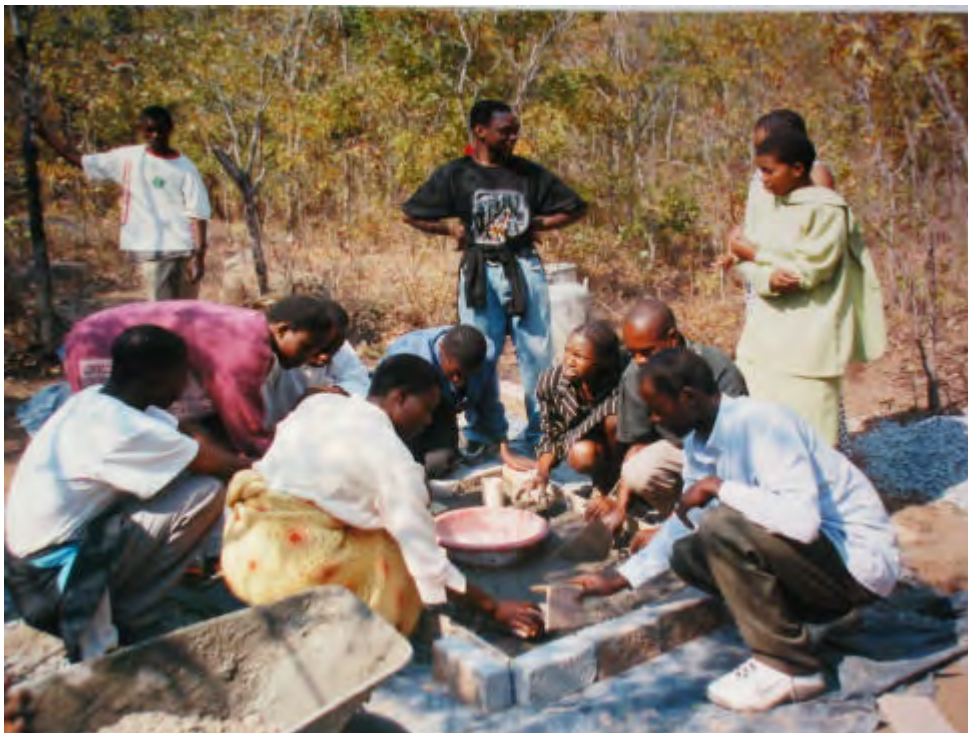
Recruits building a concrete slab at Kafunda, Ruwa
