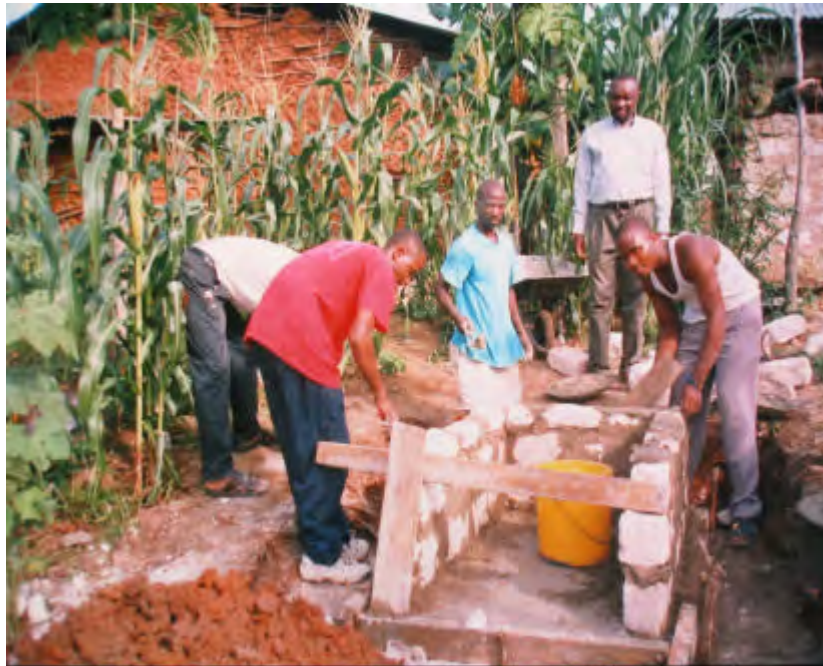
Building a single vault for the Skyloo in Mombasa, Kenya.
