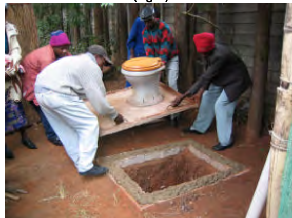
Next a thick layer of leaves is added to the base of the new pit. A layer of very weak cement mortar is added to the ring beam and the slab (in this case fitted with a plush pedestal) is lowered on to the ring beam. Finally the structure is fitted back over the slab. Good for another year.
