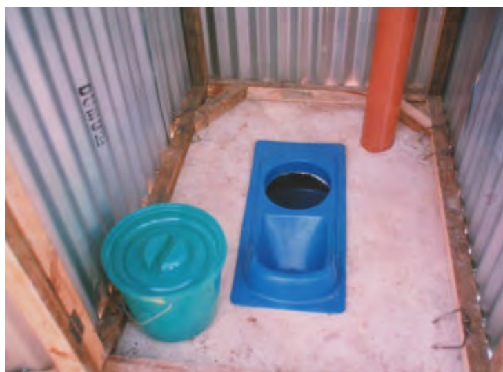
Skyloo built in Mombasa, Kenya, with external secondary composting pit chambers. This unit is fitted with a commercially made urine diverting squat plate made of tough plastic.
