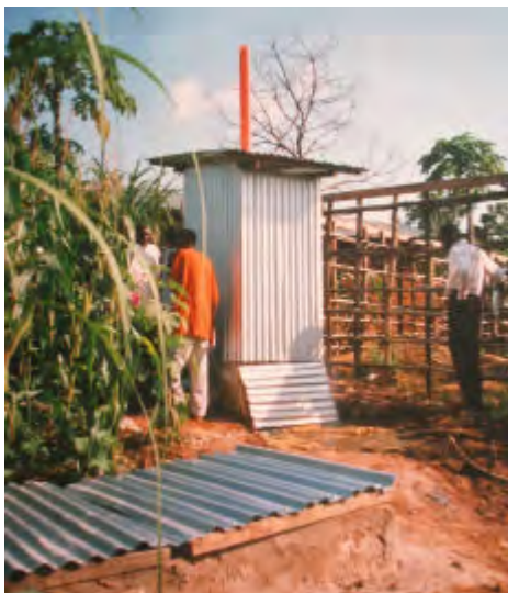
Skyloo built in Mombasa, Kenya, with external secondary composting pit chambers. This unit is fitted with a commercially made urine diverting squat plate made of tough plastic.
