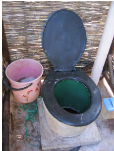
A home made hand washing device makes a popular demonstration. Also home made non urine diverting pedestal in use on a working Fossa alterna impresses people.
