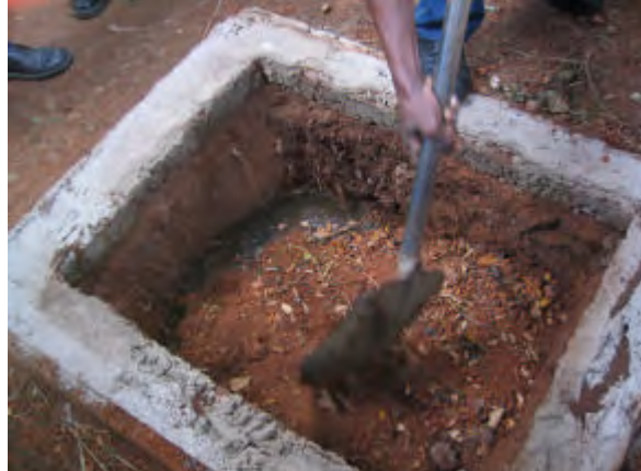
First, the structure and slab are removed from the pit which has been in use for one year. The pit contents are then covered with a good later of soil and leaves (right).
