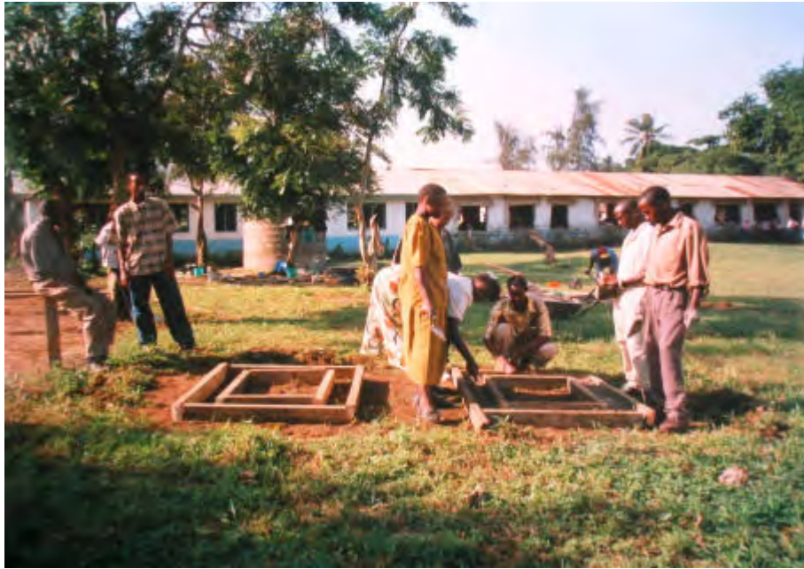
Casting ring beams at a primary school in Mombasa, Kenya
