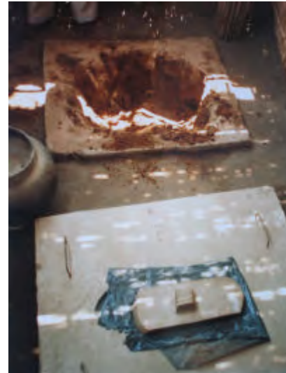
On the left - building an Arborloo near Lichinga. An Arborloo pit is just been topped up with soil and a tree planted near the foreground. On the right – the two pits of the Fossa alterna , one is partly excavated.
