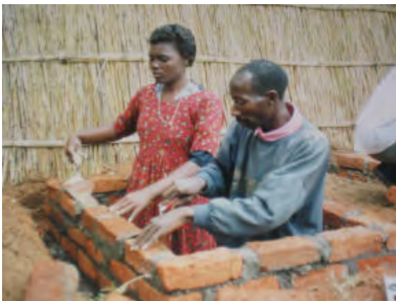
Lining the upper end of a pit in Malawi (left) and explaining the value of humus in Mozambique (right).
