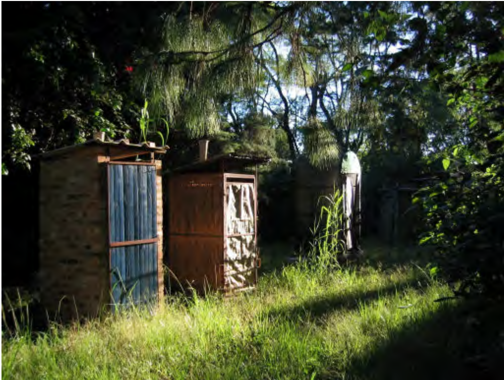
Demonstration of various ecological toilets in Harare
