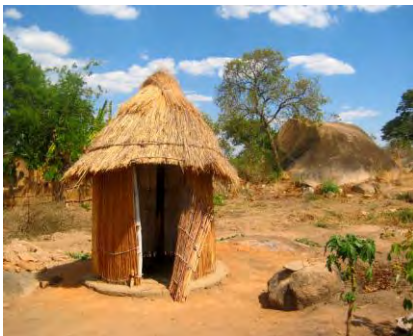
Simple Arborloo toilets built from traditional materials
