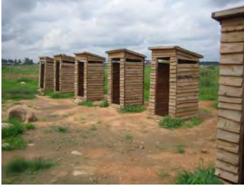
A series of Arborloo 's at a school site. Slab being removed from full pit.
