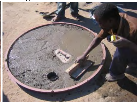
The same applies to the concrete slab. Slab diameter here is 1.2m.
