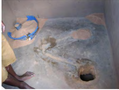
Urine diverting slabs in use in Malawi (Photos from CCODE, Malawi).
