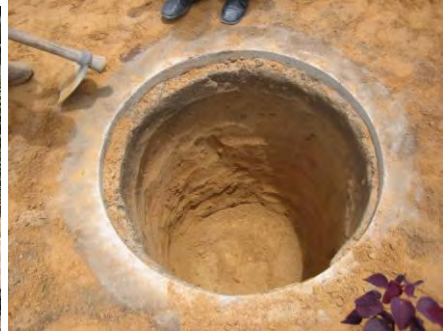
Figures 7 & 8: Digging pit inside brick ring beam.
