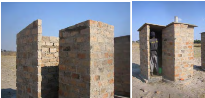
The walls are built up and roofing panels added. A short length of tubular pipe is mounted through the roof on a concrete plate (see detail elsewhere)
