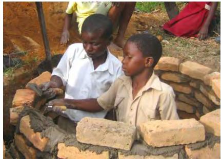
The pit is lined with bricks and corbelled at the top
