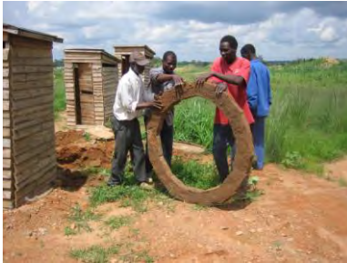
Ring being removed from pit. Pit being topped up with soil.
