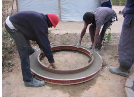
Concrete ring beams can be cast inside a brick mould or within specially made steel moulds. In this case the ring beam has an ID of 1m.
