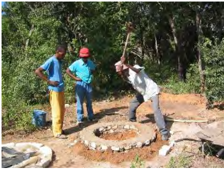
Figures 7 & 8: Digging pit inside brick ring beam.
