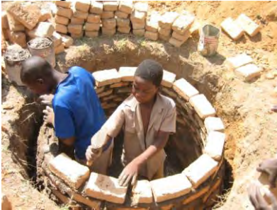
The pit is lined with bricks and the slab fitted. Space between bricks and pit wall backfilled with soil and rammed hard.
