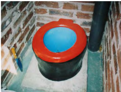
Pedestal made from concrete and a plastic bucket inside brick structure with PVC pipe. On right urine diverting pedestal fitted over pit toilet.
