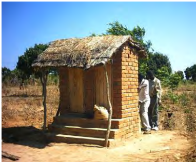
Double vault urine diverting toilet in rural Malawi (COMWASH)
