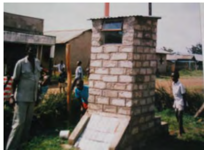
Urine diverting toilets built in Kisumu, Kenya
