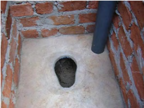
The interior can be fitted with a standard squat hole or upgraded with a pedestal. There are many ways of making a home made pedestal using cement, sand, a bucket and a seat.
