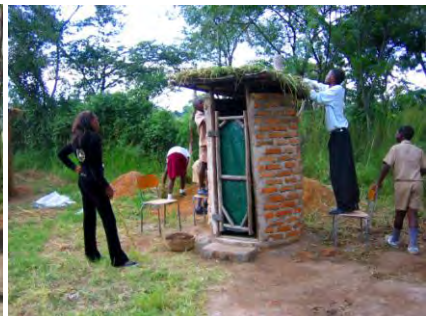
Roof, door frame and vent are added to complete the Blair VIP
