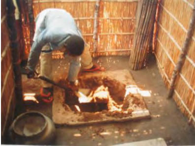
Excavating pit compost in Mozambique and Malawi
