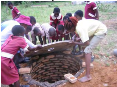
The slab is mounted over the pit and a round brick structure is built attached to a wooden door frame.
