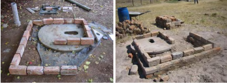
Configuration of the square spiral structure. Brick foundations are laid.
