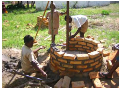
The slab is mounted over the pit and a round brick structure is built attached to a wooden door frame.
