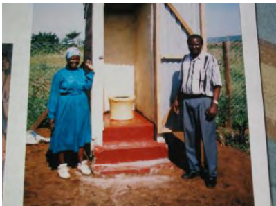
Home made toilet and urine diverting pedestal in Kenya
