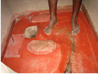
Urine diverting slabs in use in Malawi (Photos from CCODE, Malawi).
