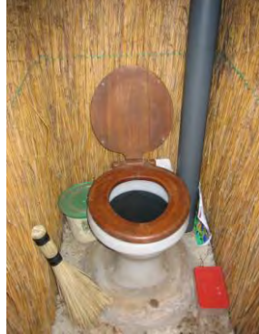
The interior can be fitted with a standard squat hole or upgraded with a pedestal. There are many ways of making a home made pedestal using cement, sand, a bucket and a seat.
