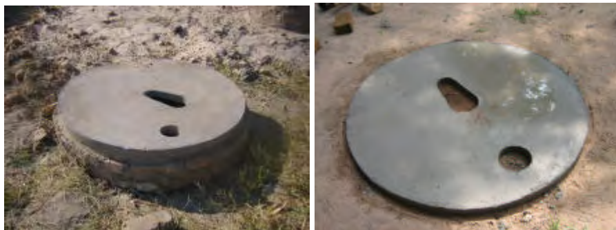
The 1.1m design (left) for tubular pipes placed inside structure. Later 1.2m design (right) used for wider range of vents. The 1.1m slab uses 10 litres of cement per slab and the 1.2m slab 12 litres of cement per slab.
