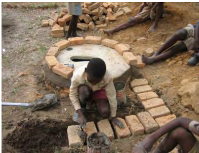
Foundations laid outside the slab and walls built on top.
