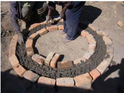
Concrete ring beams can be cast inside a brick mould or within specially made steel moulds. In this case the ring beam has an ID of 1m.
