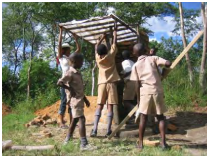
Roof, door frame and vent are added to complete the Blair VIP
