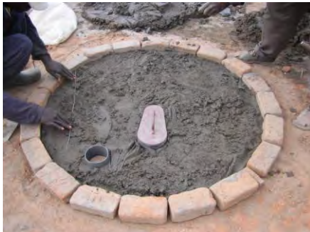
The same applies to the concrete slab. Slab diameter here is 1.2m.
