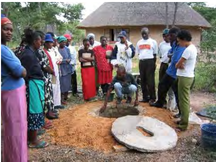
Group of trainees at Kufunda village (Ruwa, Zimbabwe) being taught how to build a simple “compost toilet.” Adding leaves to the pit.
