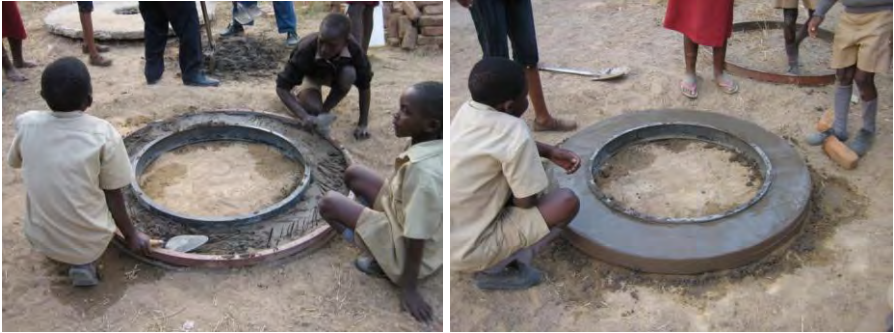
Figures 5 & 6: Steel shuttering for the ring beam
