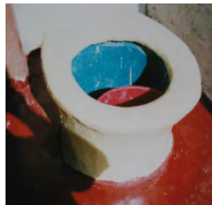
Home made toilet and urine diverting pedestal in Kenya
