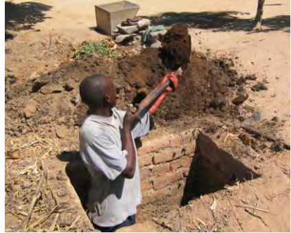
Digging out compost from a double pit compost toilet in Hatcliffe and Epworth both near Harare.
