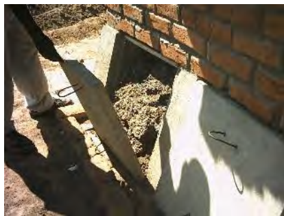
Double vault urine diverting toilet in rural Malawi (COMWASH)
