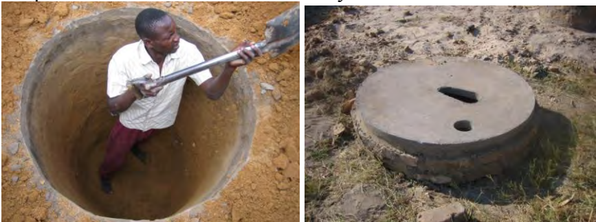
First pit being dug down to 1.5m depth. The concrete slab is then fitted and sealed with weak cement mortar.
