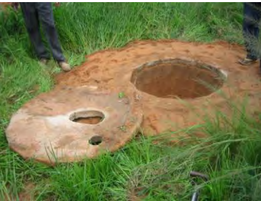
Banana being planted in compost/soil mix. The ring beam located on new site and dug down with soil being rammed around it. The slab can be fitted and the structure fitted on top. The site of a future tree in about one year.
