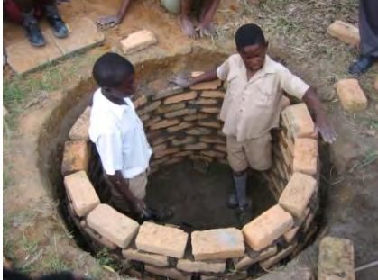
The pit is lined with bricks and corbelled at the top
