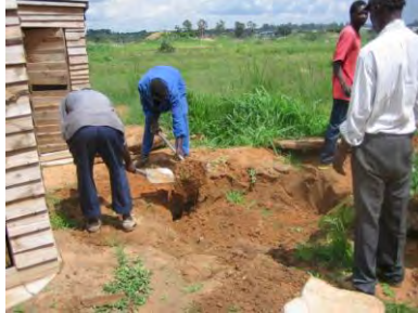
Ring being removed from pit. Pit being topped up with soil.
