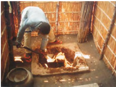
Pit contents that are not fully composted (e.g. at 6 months) can be excavated from a shallow composting pit and added to a second pit (tree pit). This is topped up with soil and a tree is planted. In this way the semi-composted material is exposed for a limited amount of time under controlled conditions.
