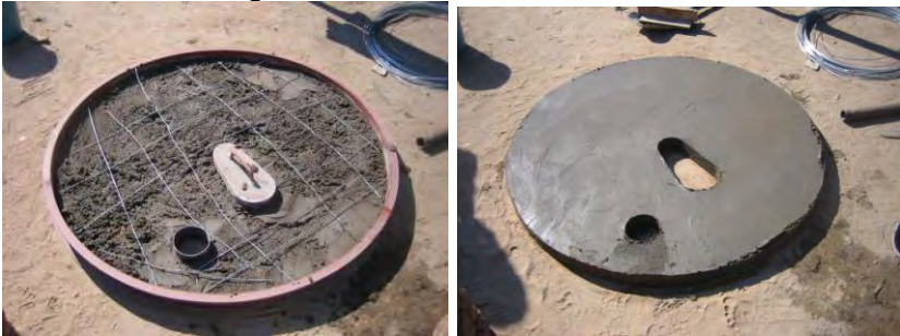
The 1.1m concrete slab
