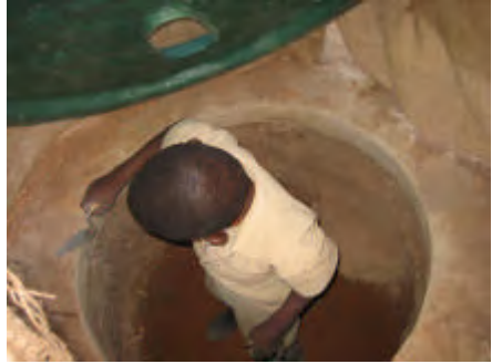
The hessian sheet is fitted all round. The hole inside the ring beam can be dug before the toilet is built or during construction.
