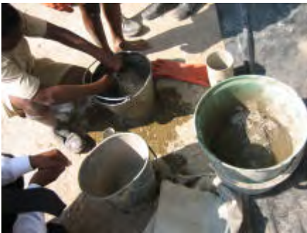
The cement paint is prepared and the hessian sheet laid on plastic sheet,
