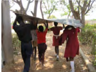
After curing the cement impregnated hessian sheet is lifted and carried to the toilet
