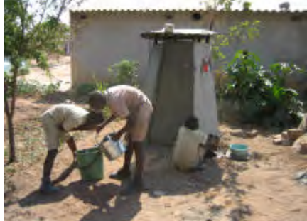
The door panel is also treated. A hand washing facility has been fitted.
