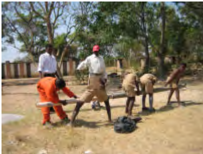
Removing folded plastic sheet and withdrawing PVC pipe
