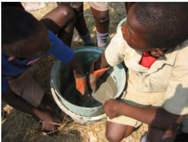
The cement mix is stirred thoroughly using rubber gloves.
