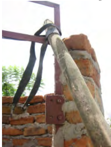
The walls of the round structure have now been built up. After a few days The two poles can now be removed as the frame is now held up by the brickwork.
