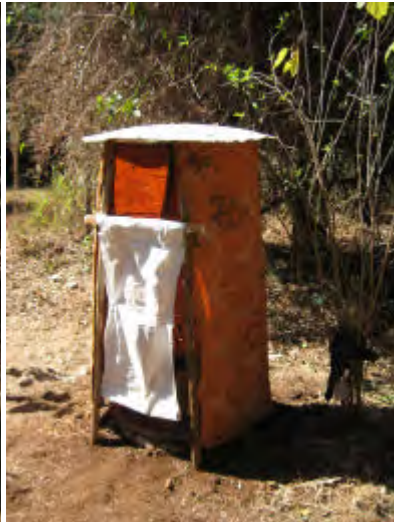
A fabric sheet is wrapped around the toilet to provide privacy. It is held in place with wire. A simple door (without hinges) has been added. In this case using poles and an opened plastic sack held at the top and weighted at the bottom.
