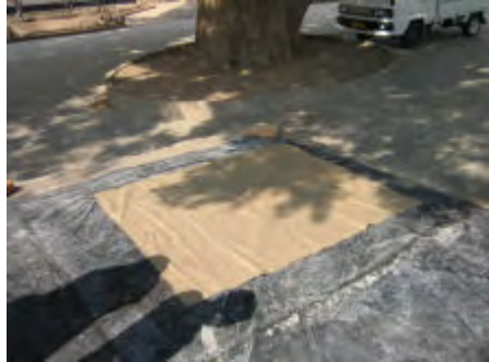
The cement paint is prepared and the hessian sheet laid on plastic sheet,
