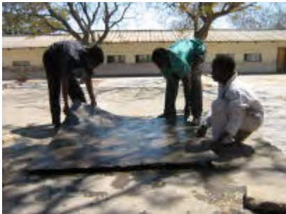
After curing the cement impregnated hessian sheet is lifted and carried to the toilet
