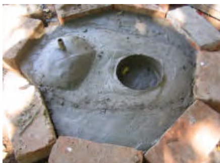
The concrete is added to a depth of 30 – 40mm. The concrete is laid carefully around the urine pipe. The concrete is allowed to cure for at least 3 days before the slab is turned over and laid on bricks, so the footrests can be added and the final surface of the slab made.
