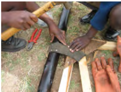
Pupils attaching the rubber hinges to the door frame and supporting pole.
