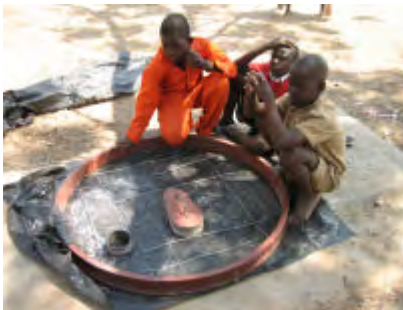
1.1m diameter concrete slab being made by school children. Steel shuttering is used and a steel mould for the squat hole.
