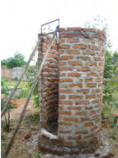
The walls of the round structure have now been built up. After a few days The two poles can now be removed as the frame is now held up by the brickwork.
