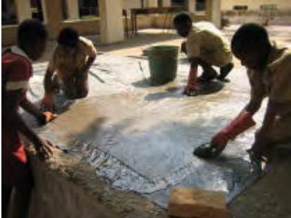
The cement paint is thoroughly rubbed into the first hessian sheet. Extra cement is added and the second hessian sheet is placed over the first. More cement paint is rubbed in all over. Then the sheet of covered with plastic sheet to cure.
