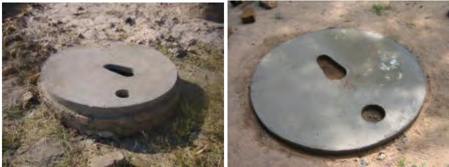
Earlier 1.1m design (left) for tubular pipes placed inside structure. Later (right) 1.2m design used for wider range of pipes. The 1.1m slab uses 10 litres of cement per slab and the 1.2m slab 12 litres of cement per slab.
