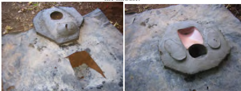
The slab can then be placed over the plastic sheet so the urine pipe enters the hole.
