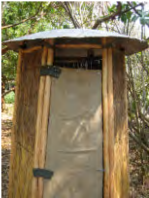
A suitably sized door panel is made and fitted the main post with rubber hinges. A hessian door covering is attached to provide privacy.
