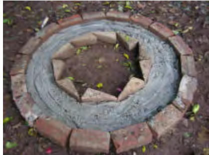
Half the concrete mix is added between the shutters and levelled off. Then two rings of 3mm wire, 3.7m long are added half way between the shutters or bricks as reinforcing.
