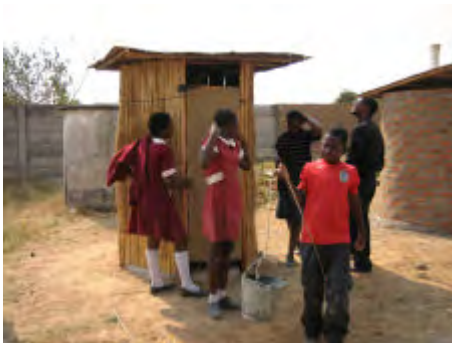
The door is added to the main “king post” with rubber tyre hinges and a door covering made (hessian).
