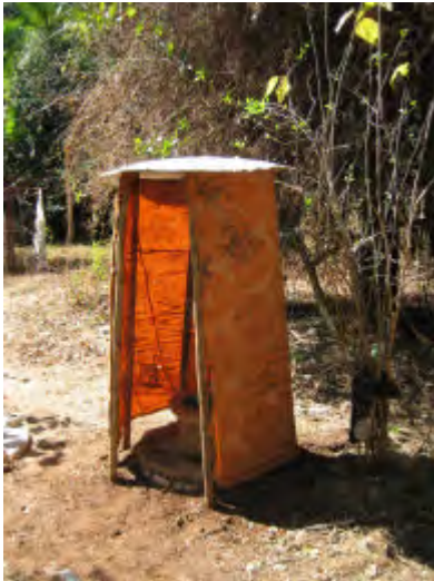
A fabric sheet is wrapped around the toilet to provide privacy. It is held in place with wire. A simple door (without hinges) has been added. In this case using poles and an opened plastic sack held at the top and weighted at the bottom.
