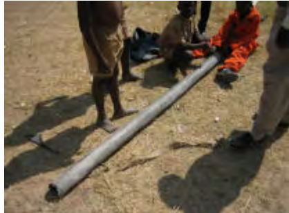
Removing folded plastic sheet and withdrawing PVC pipe
