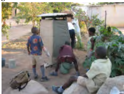
All the panels are treated with the liquid cement which is applied with a large brush.
