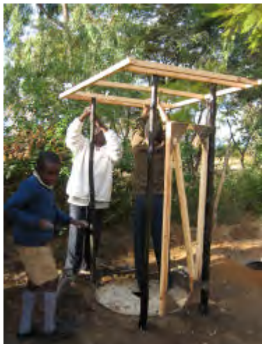
Attaching the frame to the simple treated gum poles structure. And adding the cement filled hessian sheet to the frame.
