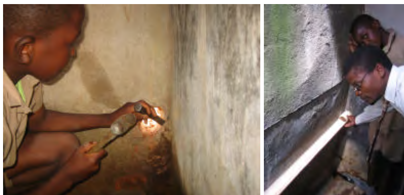
The PVC pipe is used as a urine collector and attached to the existing wall of the urinal. The pipe was 2.5m long made from 75mm PVC pipe. A section of 1.7m was cut out to form a channel in which the urine will flow. A hole is made in the external wall of the urinal and the pipe is placed along the existing urinal wall leading out through the wall to fit over the tank outside.
