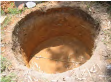
Dig hole and assemble bricks
