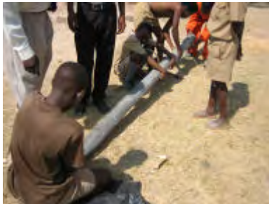
Removing folded plastic sheet and withdrawing PVC pipe
