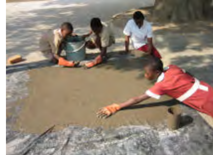
The cement paint is thoroughly rubbed into the first hessian sheet. Extra cement is added and the second hessian sheet is placed over the first. More cement paint is rubbed in all over. Then the sheet of covered with plastic sheet to cure.
