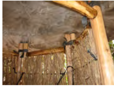
A domed cement impregnated hessian roof is added on top and can be wired in position for security.
