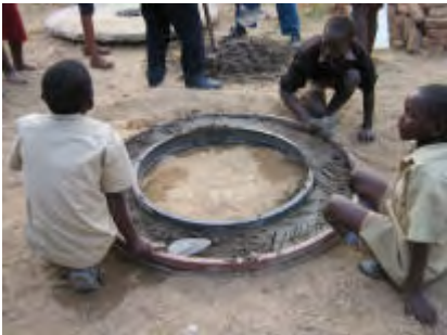
Half the concrete mix is added between the shutters and levelled off. Then two rings of 3mm wire, 3.7m long are added half way between the shutters or bricks as reinforcing.
