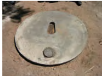
1.2m slab with vent hole filled in (temporarily) or with concrete cover.
