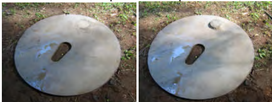
1.2m slab with vent hole filled with weak cement mortar. This can be used as a start up slab. When the upgrade takes place and a pipe is built or fitted, the weaker mortar is knocked out exposing the vent hole in the slab. The alternative (right) is to make a small concrete cover and mortar in place over the vent hole.
