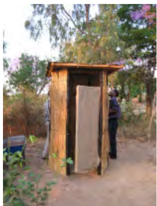
The roof sheet is attached to the roof sheet using small nails. The roof frame can either be nailed or wired to the supporting poles.
