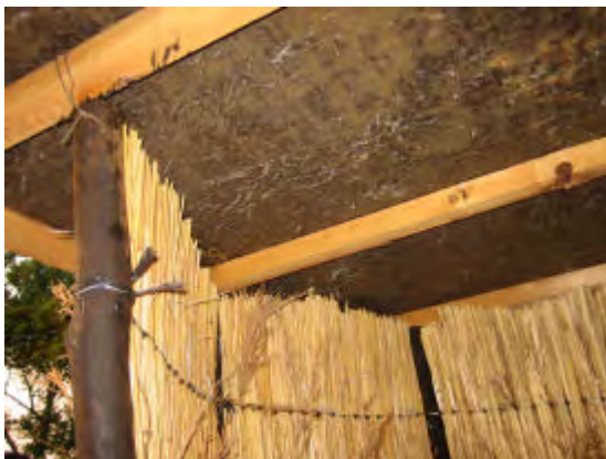
The roof sheet is attached to the roof sheet using small nails. The roof frame can either be nailed or wired to the supporting poles.
