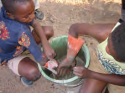
The cement mix is made in a large bucket and thoroughly mixed using long rubber gloves.
