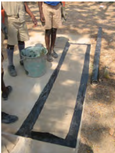
The hessian sheet is then cut 2 pieces measuring 2.3m long and 40 wide. The first sheet is laid on plastic. The application of the cement paint begins.
