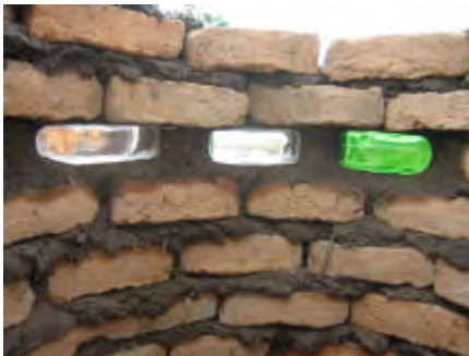
Photo showing glass bottles in wall. The full height of the superstructure is about 19 courses of bricks.
