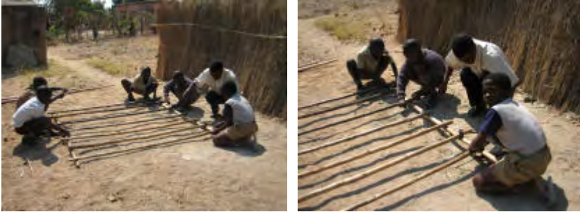
Binding the roof timbers with thatching twine
