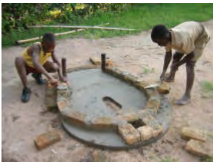
The bricks are laid in the mortar so they join up with the door posts in a gentle curve (horseshoe shape). A second course of bricks is laid for the vent pipe. The brick walls and pipe are then extended upwards so the final height of the wall is about 1.8m and the vent 2.3m.
