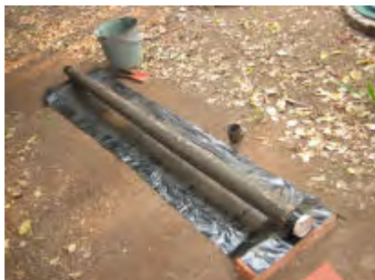
Further stages of pipe construction
