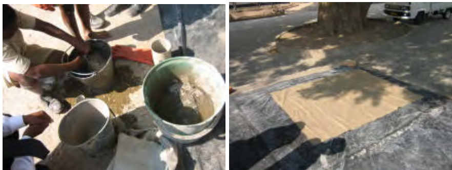
The cement paint is prepared and the hessian sheet laid on plastic sheet,
