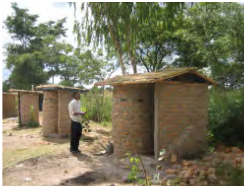
Roof in position
