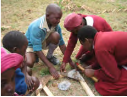
Pupils putting together the door frame with triangular pieces of plywood and nails.
