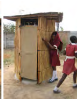
The door is added to the main “king post” with rubber tyre hinges and a door covering made (hessian).
