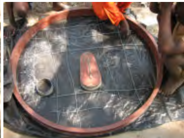
1.1m diameter concrete slab being made by school children. Steel shuttering is used and a steel mould for the squat hole.
