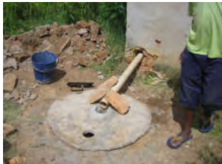
The base of the tank is also plastered with the mortar. The lid is then fitted with mortar being laid on the upper brickwork in which the lid is embedded. The pipe is laid in position to check that the end lies over the tank opening
