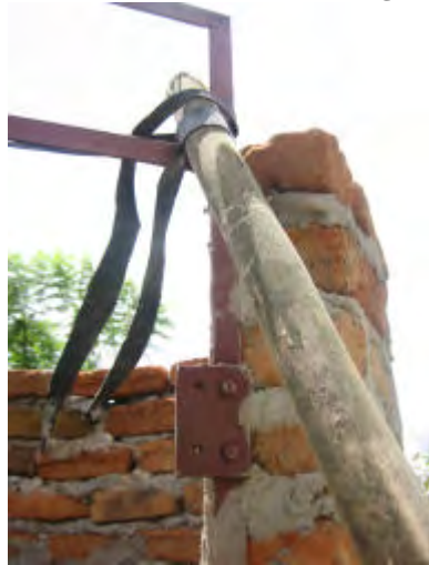
The walls of the round structure have now been built up. After a few days The two poles can now be removed as the frame is now held up by the brickwork.
