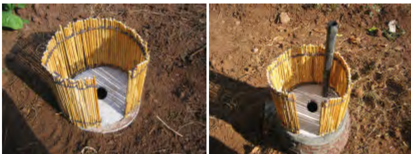
House without vent and with a vent. When a vent is fitted without a roof, flyscreen and semi-darkened structure, odours will be removed but there will be no fly control. Many types of model superstructure can be made.
