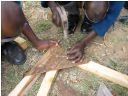
“Brandering” timber was used to make the door. The timber lengths were held together using triangular shaped pieces of plywood.
