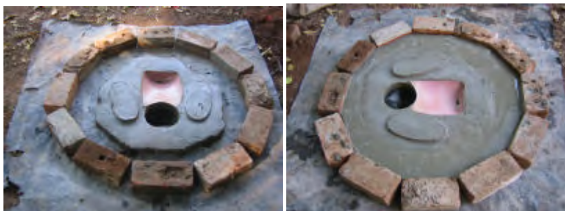
A circle of bricks is laid down around the slab to the required size. This is then filled with concrete with some reinforcing wire inserted. It is left to cure. This urine diverting slab offers a clean non absorbent surface for urine collection, which can be made at low cost.
