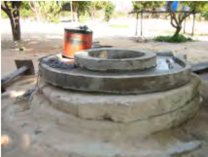
The new well apron is laid on the exiting well slab and cement bonded in position
