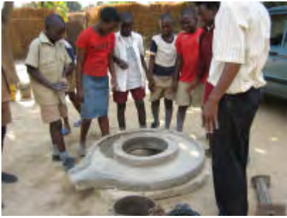
The new well apron is set in position so that the water run-off channel will carry water slightly down hill to a seepage area planted with a tree
