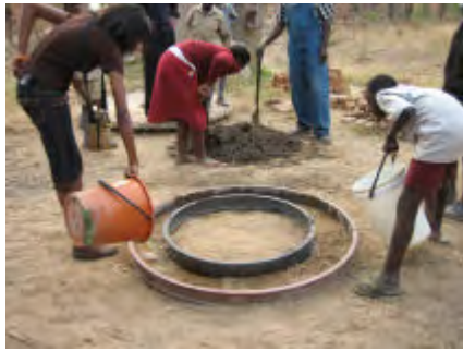
A mix of 10 litres of Portland cement and 60 litres of river sand is prepared. The soil on the ground within the ring beams is wetted down.
