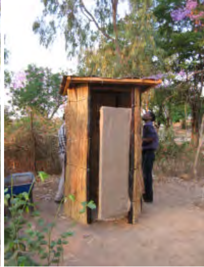
The roof sheet is added to the roof frame and secured with small 25mm nails
