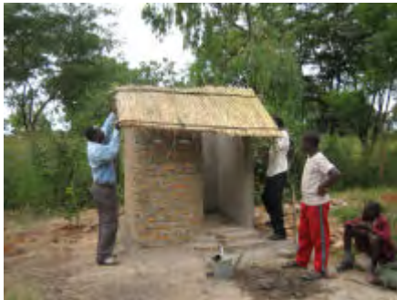
Fitting the front panel to the toilet. Additional bricks are added to the walls of the structure to support and raise the centre of the roof to give it a slope. Grass roofs can be smart, although they require more maintenance than asbestos, tin or concrete roofing sheets.
