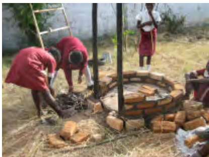
The brickwork is then built up course by course.
