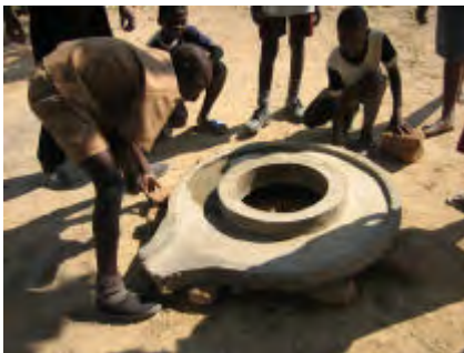
After a week of curing (being kept wet at all times) the apron is moved on to the existing well slab
