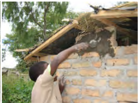
Fitting the front panel to the toilet. Additional bricks are added to the walls of the structure to support and raise the centre of the roof to give it a slope. Grass roofs can be smart, although they require more maintenance than asbestos, tin or concrete roofing sheets.
