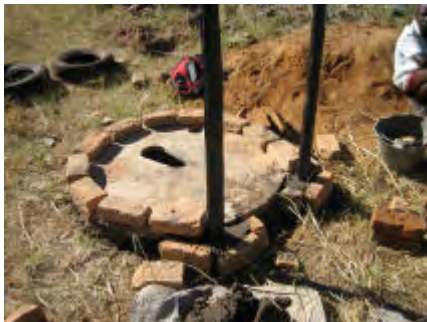
The second pole is placed in position. Once correctly placed the holes are filled with stones and soil which is rammed hard in place.
