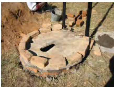
The bricks are then laid in a circle to form the horseshoe shape. Cement mortar is made. This can be 16 parts pit sand to 1 part cement. The bricks are laid with plenty of mortar between them.
