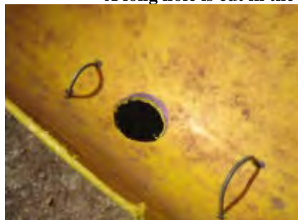
A hole is also cut with a sharp knife in the cut section of bucket at the lowest part where the urine will collect
