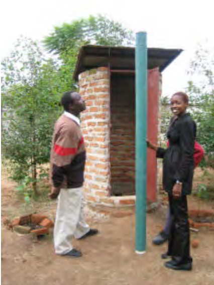
This pipe is a new unit on the market and is being field tested. It is about half the cost of a PVC pipe. A length of PVC pipe is fitted at both ends.
