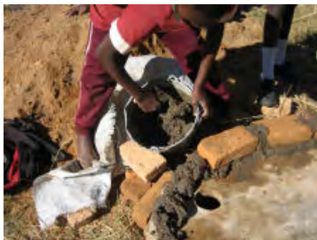
The bricks are then laid in a circle to form the horseshoe shape. Cement mortar is made. This can be 16 parts pit sand to 1 part cement. The bricks are laid with plenty of mortar between them.
