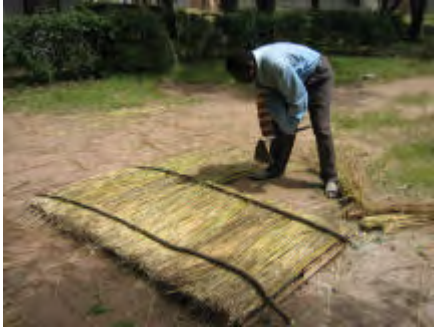
Finishing off one roof panel. Carrying the roof panel to the toilet.
