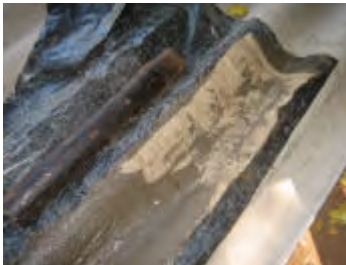
The hessian cement water run-off channel 1.5m long
