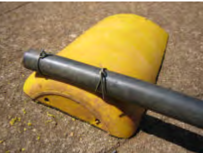
Small holes are then drilled into the bucket, through which wires are massed to secure the polyethylene pipe. Urine will fall into the urine collector and then through the pipe and out of the slab.
