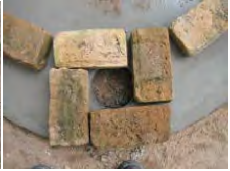
The finished toilet floor before mortaring the bricks in place. The arrangement of the brick pipe around the 140mm diameter hole.
