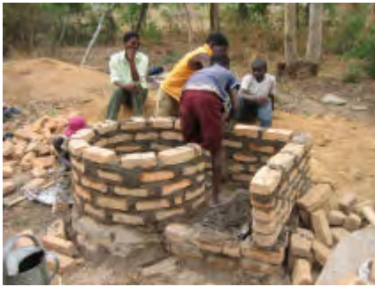
The brickwork continues upwards
