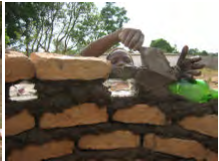
At about the 15 th course some glass bottles are introduced into the brickwork. These will later act as windows allowing a little more light into the toilet house. They are cement mortared in position and the brickwork then continues upwards.
