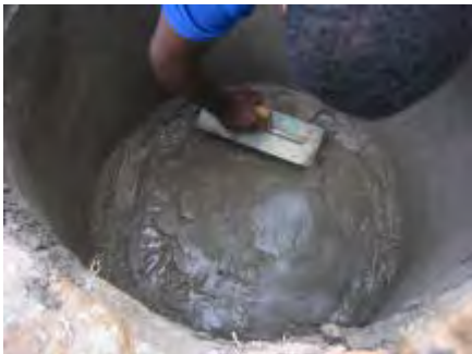
The base of the tank is also plastered with the mortar. The lid is then fitted with mortar being laid on the upper brickwork in which the lid is embedded. The pipe is laid in position to check that the end lies over the tank opening
