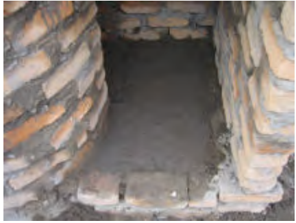
Some cement mortar is then laid on the soil placed
