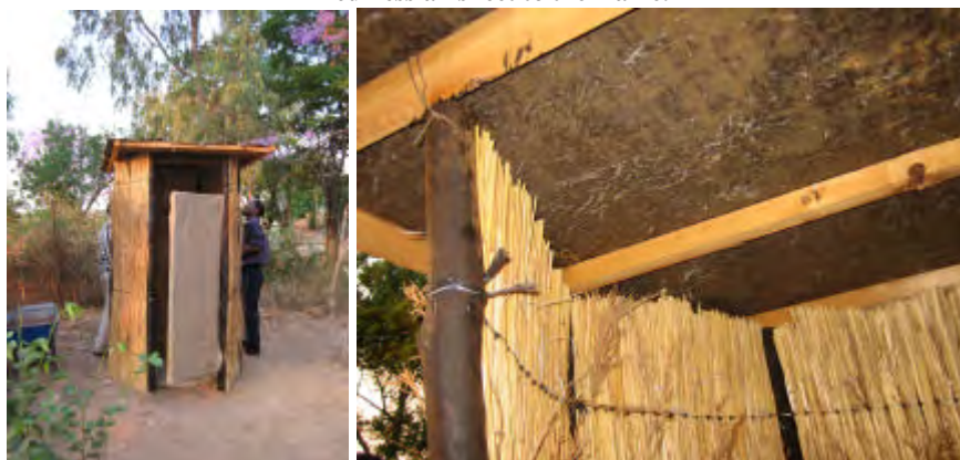
The roof sheet is attached to the roof sheet using small nails. The roof frame can either be nailed or wired to the supporting poles.
