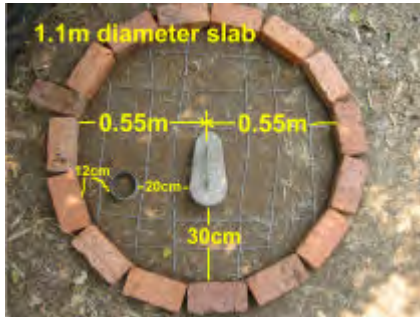
Figures 10 & 11: Brick mould for slab showing the dimensions for locating squat and vent pipe holes and also position of the 3mm wire reinforcing. Diagram showing layout of wire reinforcing.
