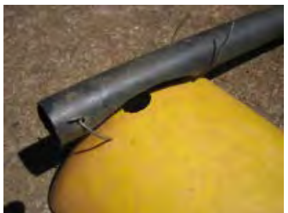
Small holes are then drilled into the bucket, through which wires are massed to secure the polyethylene pipe. Urine will fall into the urine collector and then through the pipe and out of the slab.
