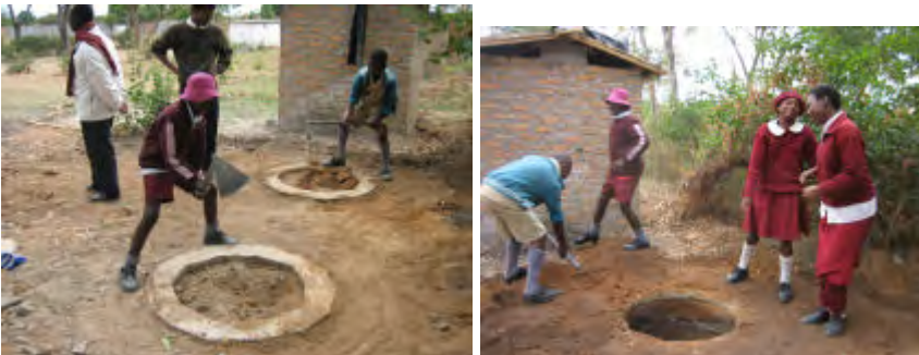
Lay 2 ring beams and dig 2 pits inside
