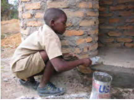
Some cement mortar is then laid on the soil placed
