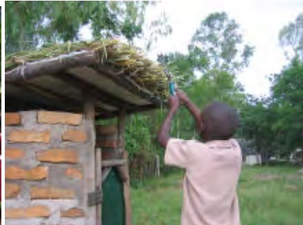
Grass this then laid over the plastic sheeting and this is secured by laying reeds across the top of the grass. It is possible to fit other types of roof to a brick structure such as tin, asbestos or ferro-cement. A hole is made in the roof to fit the vent pipe once it has been made.
