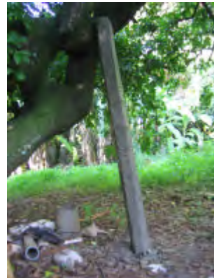
A section of the cloth is coated in a strong cement and sand slurry to demonstrate the method. The full length pipe completed.
