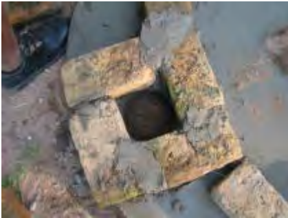
Using a weak economical cement mortar mix (20 parts pit sand to 1 part PC15 cement) the bricks of the vent and walls are bonded together. If traditional anthill mortar is used for the walls, the pipe should still be mortared with cement mortar.
