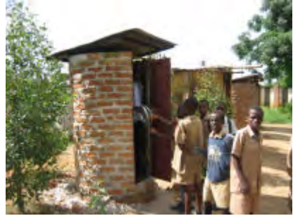
The roof is then mounted on the toilet and wired in place.
