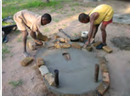
Using a weak economical cement mortar mix (20 parts pit sand to 1 part PC15 cement) the bricks of the vent and walls are bonded together. If traditional anthill mortar is used for the walls, the pipe should still be mortared with cement mortar.
