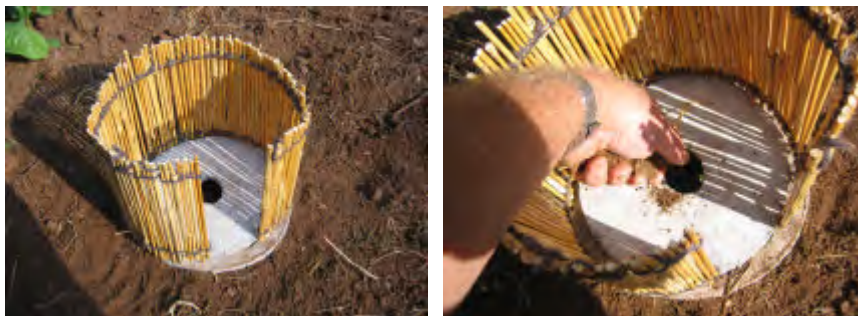
The simple structure is now fitted and the Arborloo put to use
