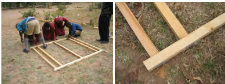
Making the roof frame
