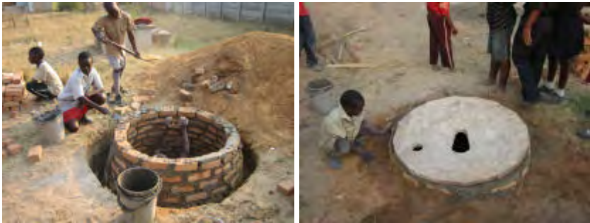
The original pit and slab
