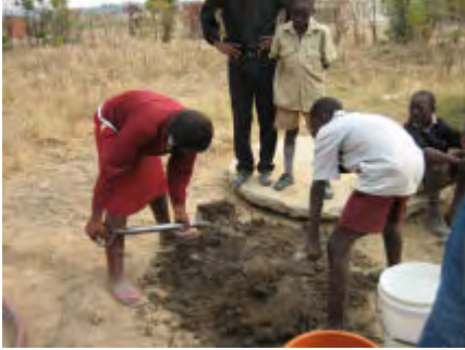
A mix of 10 litres of Portland cement and 60 litres of river sand is prepared. The soil on the ground within the ring beams is wetted down.
