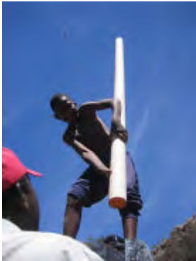
The cement mortar is allowed to cure overnight. The pipe is then removed with a twisting motion and completely removed from the toilet. Next the plastic sheet is twisted and pulled out of the cement plaster tube.
