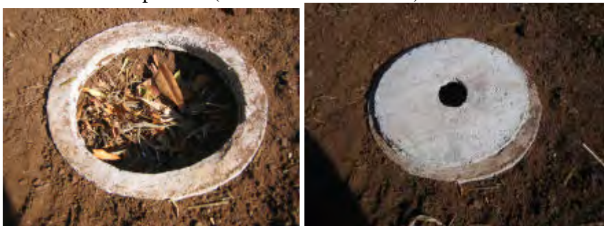
The ring beam has been cast on ground allowed to cure and a hole dug down inside. The slab has been fitted.
