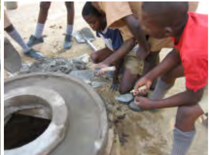
The new well apron is laid on the exiting well slab and cement bonded in position
