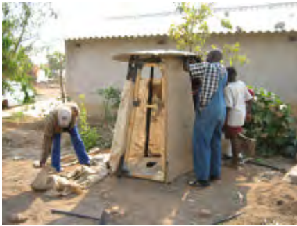
The hessian sheet is fitted all round. The hole inside the ring beam can be dug before the toilet is built or during construction.
