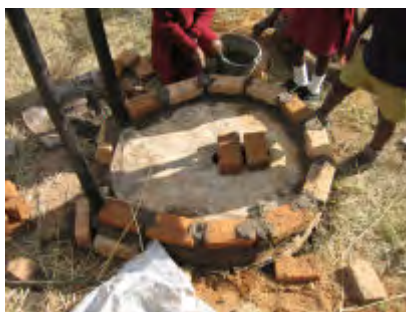
The brickwork is then built up course by course.
