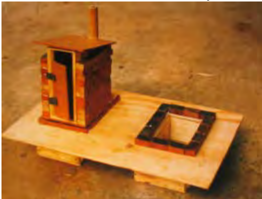
A model of a Fossa alterna with square slab and ring beam – 2 versions!
