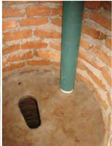
This pipe is a new unit on the market and is being field tested. It is about half the cost of a PVC pipe. A length of PVC pipe is fitted at both ends.
