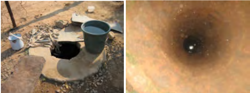
The existing well on the surface and down below
