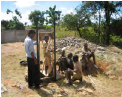
The second pole is placed in position. Once correctly placed the holes are filled with stones and soil which is rammed hard in place.
