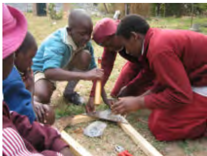
“Brandering” timber was used to make the door. The timber lengths were held together using triangular shaped pieces of plywood.
