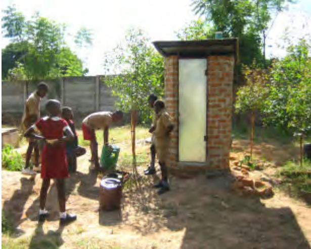
The completed toilet.
