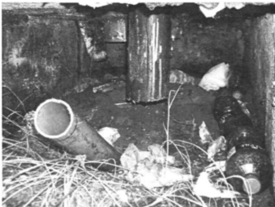
Figure 3.2.1 Taking a sample through the rear opening of a vault. The sampling tube is the PVC pipe in the foreground of the picture.
