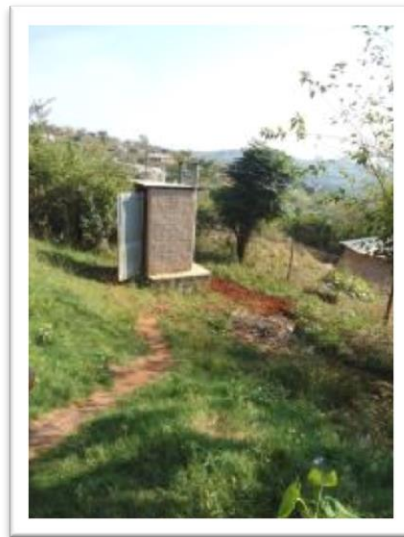
Figure #16: A urine diversion VIP at a single family residence in Mzinyathi
