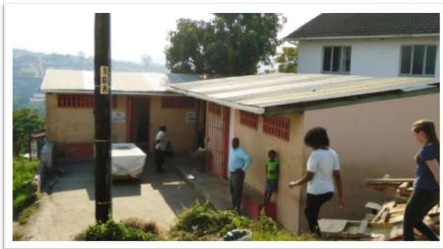
Figure # 18: A six-year-old ablution block that hosts 81 families. The block is run by a caretaker who transformed it into a social gathering place. The caretaker implemented a billiards table (covered by white cloth) and runs a store from his shack, just across from the block.
