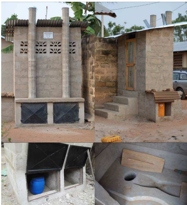
Fig. 7: Domestic EcoSan latrine (source: E. Albert, 2014)
