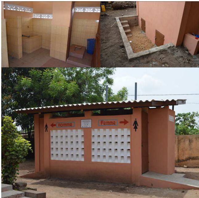
Fig. 9: Public EcoSan latrines in the city council of Lokossa (source: A. Dubois, 2014)
