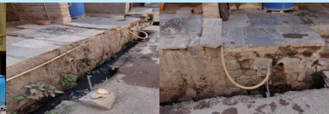
Septic tanks tops are sealed
