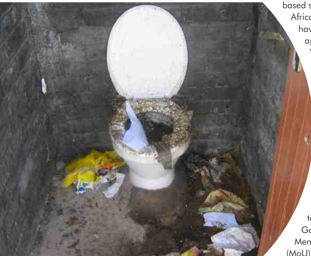
Photograph of school toilet in the Eastern Cape Province. Photo by Oliver Iwe (Amanz'abuntu).
