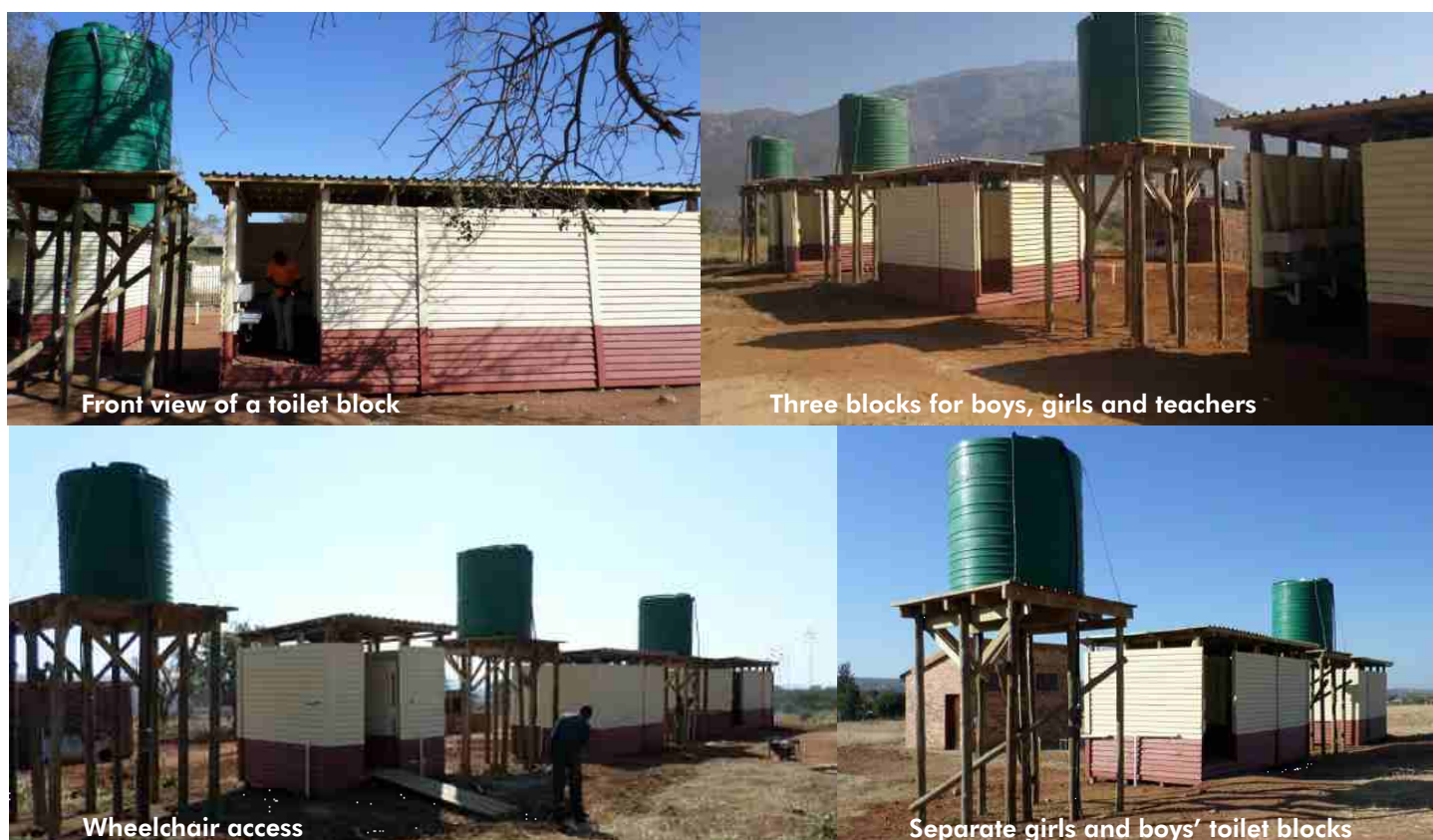
Fig.12. Timber frame toilets housing low flush units.
