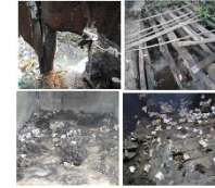
Fig. 5 Photos showing full pit latrines & the residents were forced even to use the slab for defecation
