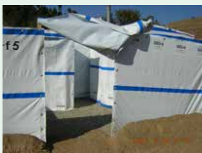
Looking into the screened washing and bathing unit through the main entrance
