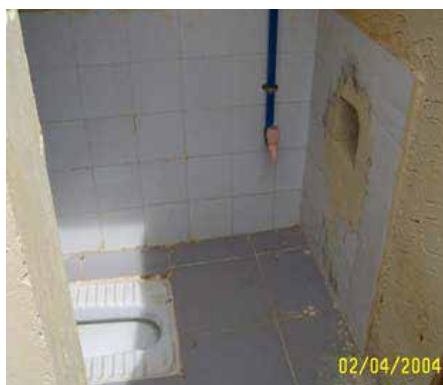
Disposal shoot inside the latrine
