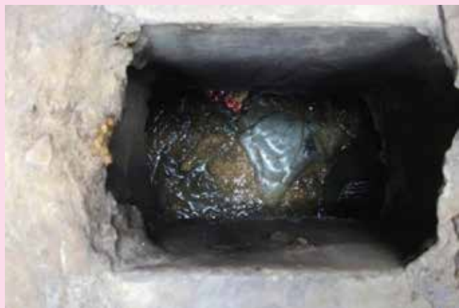
Solid waste that has been disposed of in a pit latrine (Photo: Belen Torondel/LSHTM)
