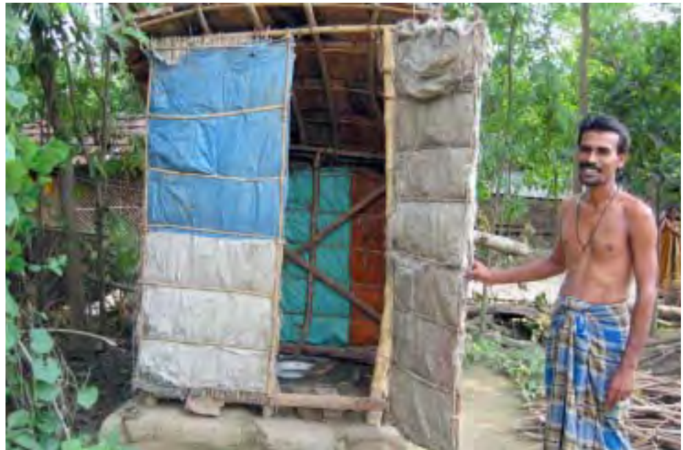
ABOVE Use of bamboo and plastics in making the super structure while the sub structure is strong and perfect. Vidyasagar colony, Kalyani, West Bengal India.
