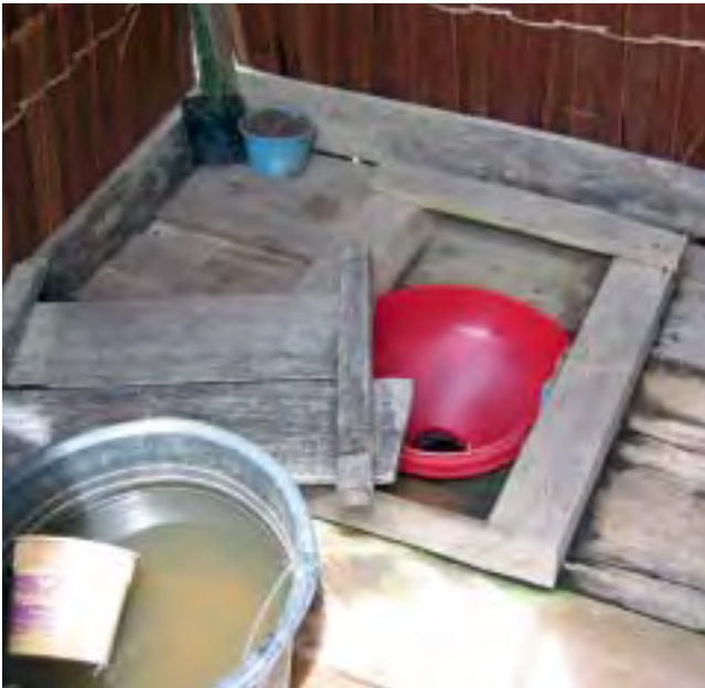
ABOVE A latrine constructed in South Sumatra, Indonesia. A woman used some household materials to construct a makeshift latrine in order to comply with the communities decision to go ODF, while her husband was away.
