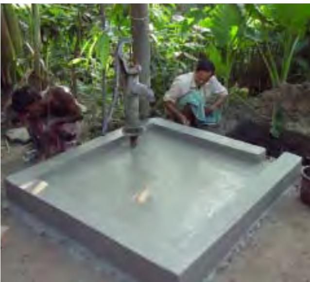
ABOVE AND RIGHT Community women of Vidyasagar colony of Kalyani The Municipality in West Bengal, India, decided to pave the base of all the 69 hand pumps in their colony and construct cemented platforms to avoid accumulation of waste water, garbage and filth around the drinking water source. Municipality gave them some unused brick-bats the rest was done by them. All this happened within two months of achieving of ODF status. This was the first slum to attain ODF status. Within a year all the 52 slums in the Municipal town were declared ODF.
