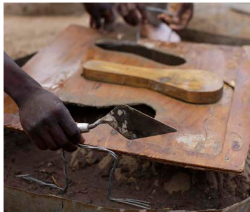
Promoters making a latrine slab, Chikomplazi village, Mzuzu, Malawi. Credit: WaterAid/Layton Thompson.
