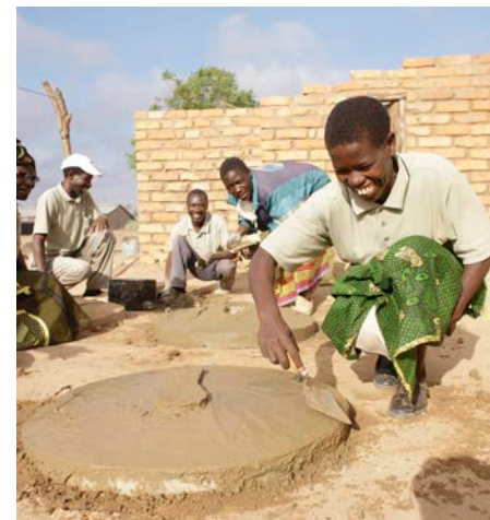
Elifa Mwaungulu, building a latrine slab, Chikompulazi village, Mzuzu, Malawi. Credit: WaterAid/Layton Thompson.
