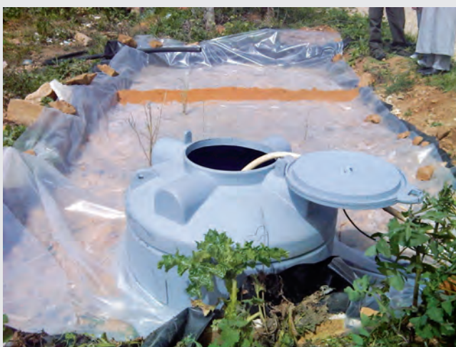
Figure 6: Treatment trench at Jerash, Jordan
