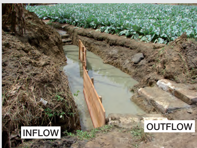
Figure 4: Interconnected pond with hardwood baffle.
