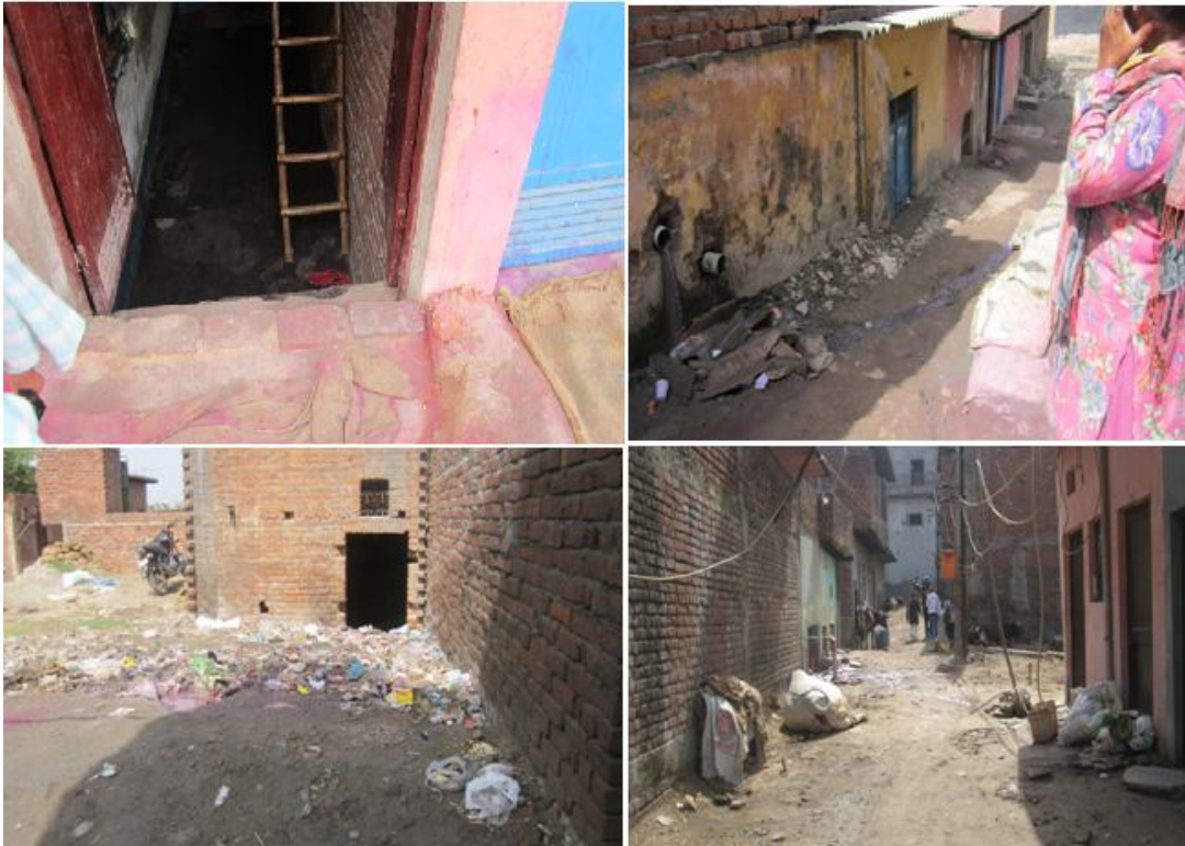
(Picture 1: Houses Built on Low Land in Saboli Khadda)
