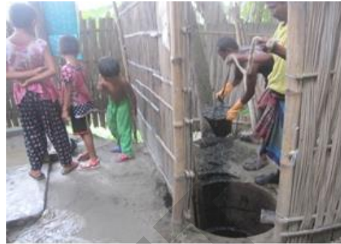
Photograph 2. Manual pit emptying by private sweepers
