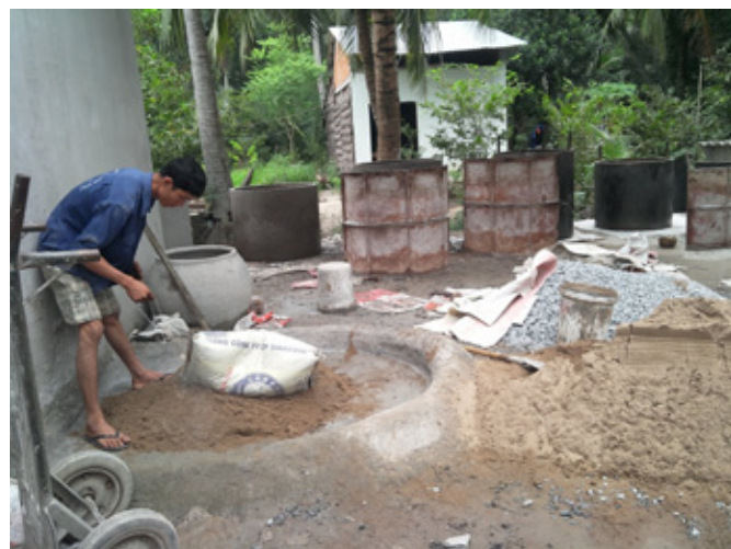
FIGURE 2 SMALL-SCALE ENTERPRISE MANUFACTURING CONCRETE RINGS IN THE MEKONG
