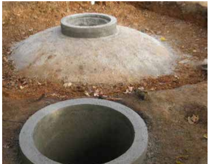
Figure 12: The finished chinese dome type biodigester is barely visible when completed.
