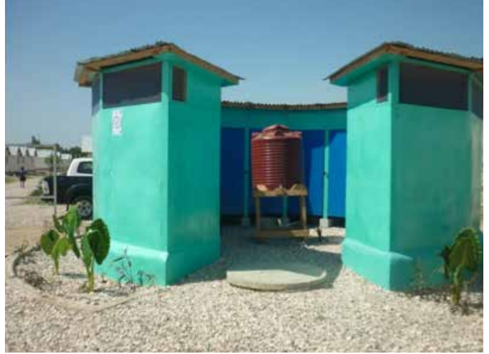
Photo VR_8: Emergency biodigester in transitional camp Santo 17.
