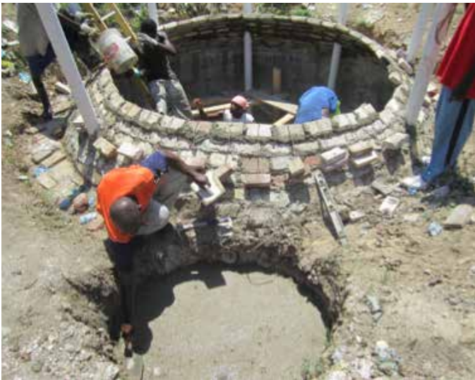
Figure 11: Biodigester construction did improve during the dissemination period.
