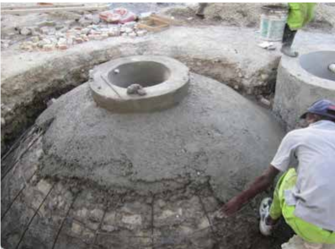
Photo VR_9: Reinforcing of biodigester dome.
