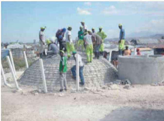
Photo VR_3: Training of Viva Rio Biogas Technicians, dome strength.
