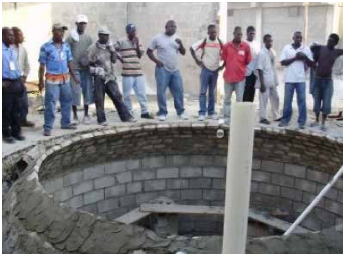
Photo VR_1: Initial training of Viva Rio Biogas Technicians.
