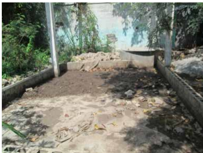
Figure 17: Sludge Drying bed used as a pre-cursor to compost production, Kay Nou. (TF 001).
