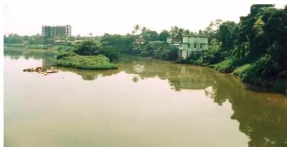
Figure 1: Water supply intake at Periyar river (CDP Kochi 2006)
