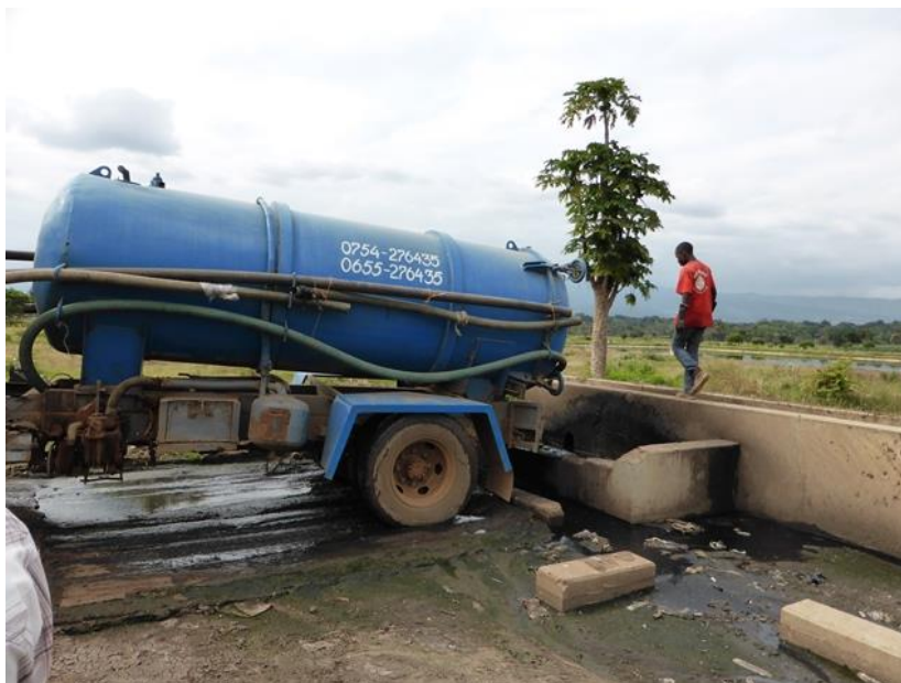
Fig. 3: Privately operated FS truck discharging at Mabogini wastewater treatment ponds (Source: L. Roeder 2015)
