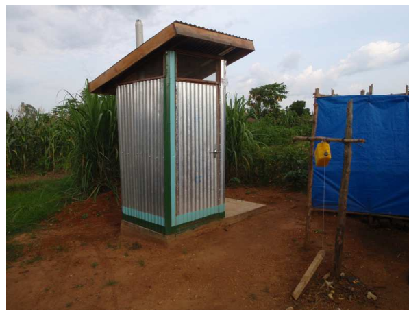
Figure 1: Pilot pit latrine provided by DUWSS (Source: GIZ 2015)
