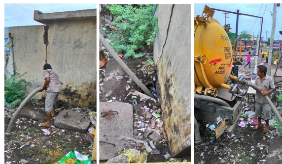
Figure 1: Emptying process of septage from community toilet (Source: Rahul/CSE, 2015)
