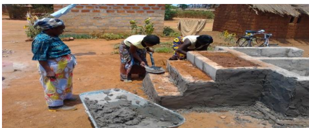
Figure 5: Capacity building of Madimba women in dry sanitation (Source: NECOS verification
