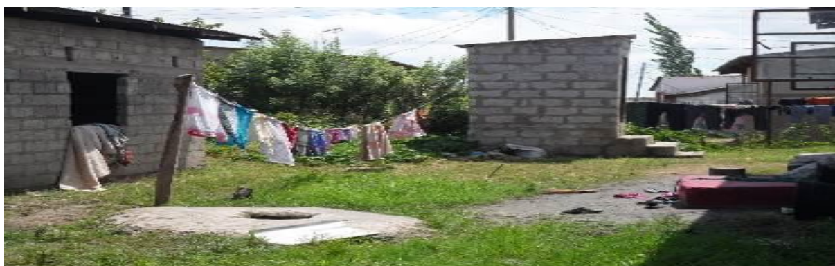
Figure 2: Madimba Community Latrine constructed in proximity with shallow water well.
