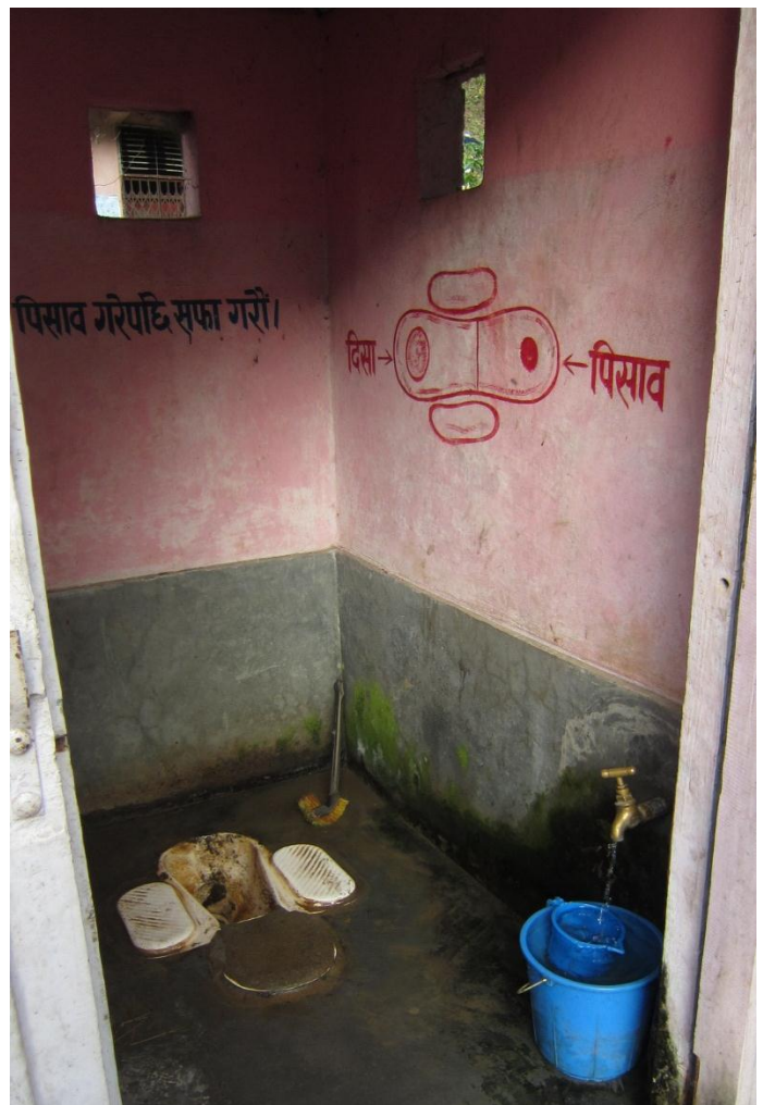
Photo : Blocked urinal of EcoSan Toilet at Syngja (Photo: RWSSP-WN Phase II)
