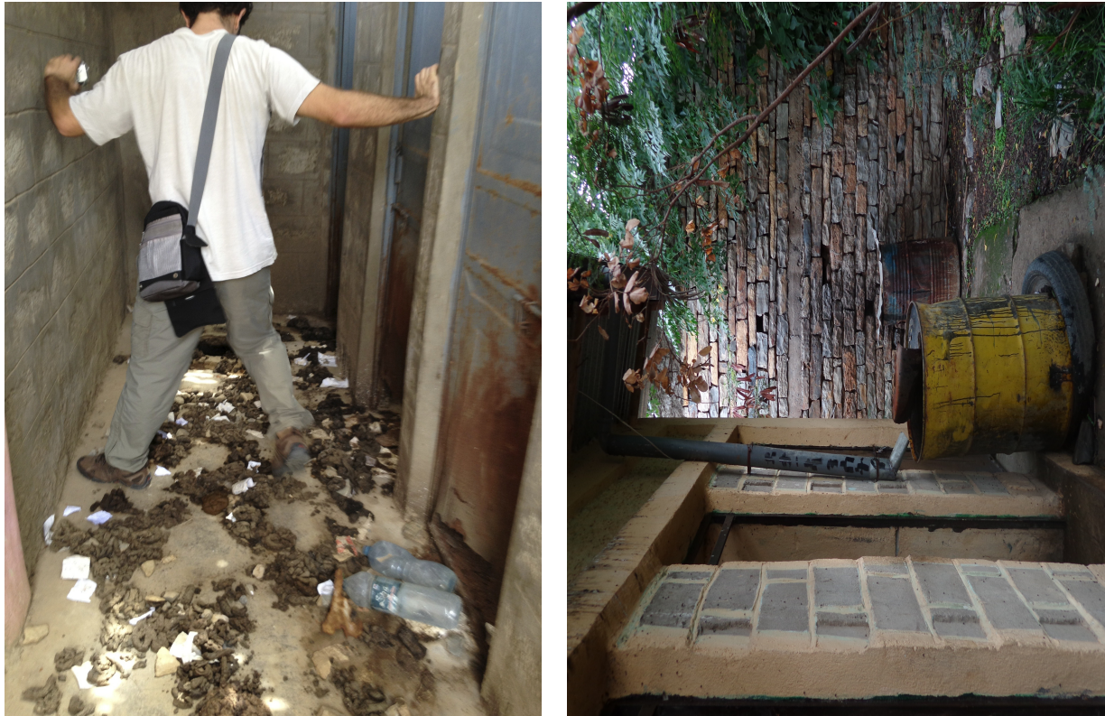
Figure 4: Poor hygienic conditions (left) and rainwater collection from rooftops (right).
