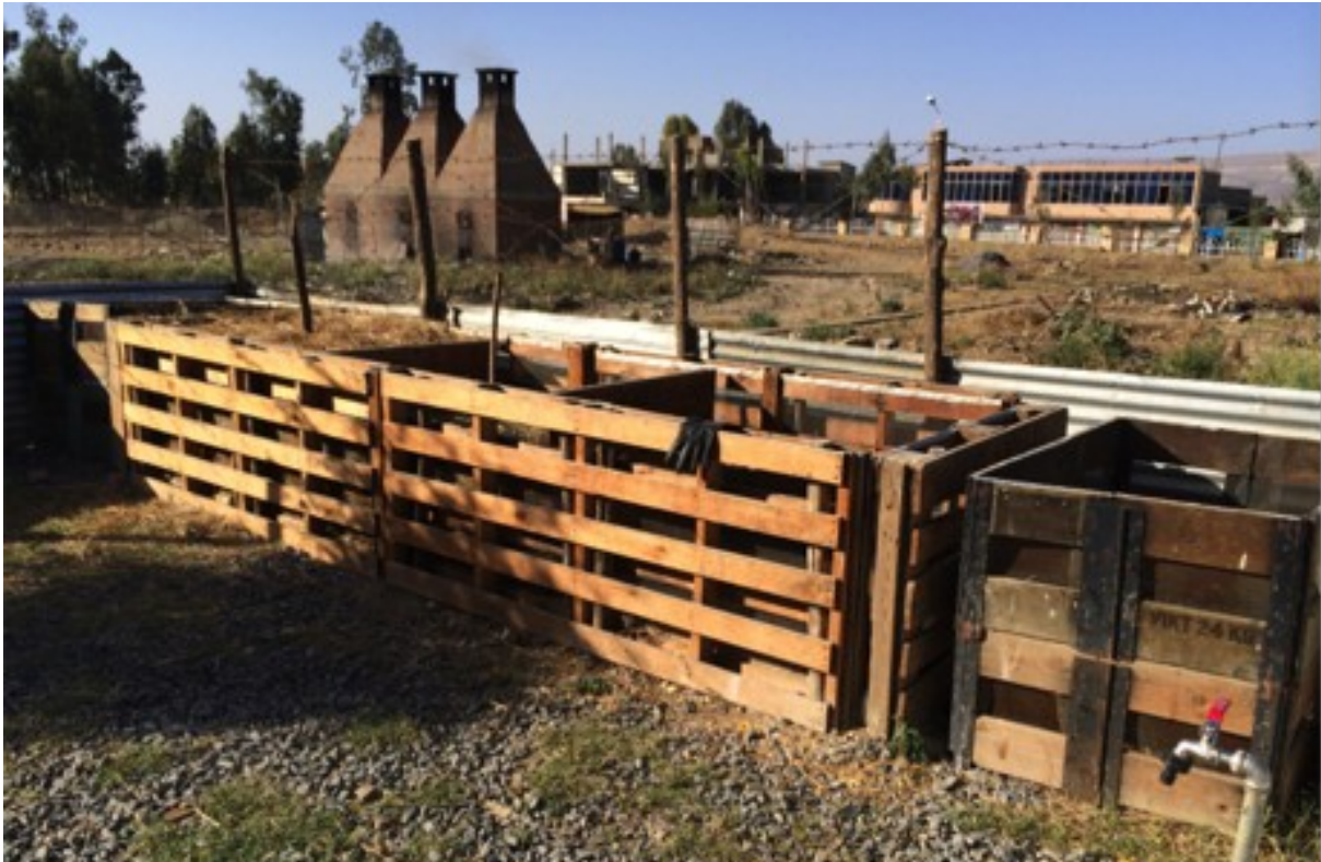
Figure 13: Composting area adjacent to the toilets.
