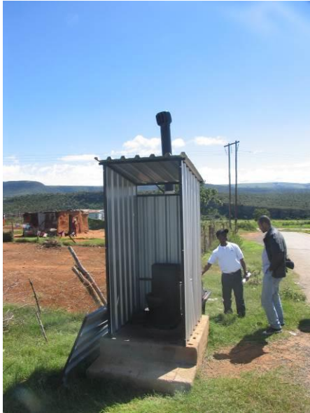
Figure 1 and 2. One of the composting toilet models used in the Makana villages. Photo by Javier López-Murcia.
