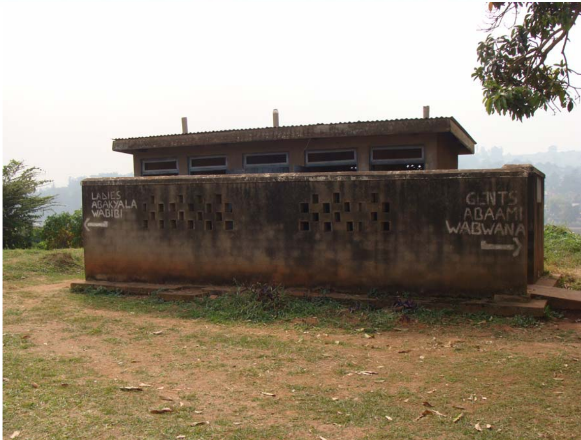
Uganda; toilet blocks outside
