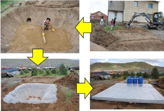
Figure 3: System construction stages
