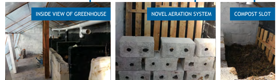
FIGURE 3-22 ECO-TOILET ORIENTED SEMI-CENTRALIZED GREENHOUSE COMPOSTING UNIT.
