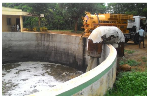
Figure 1: Private emptier discharging septage in to sewage pumping station (Source: Bhitush/CSE, 2015)
