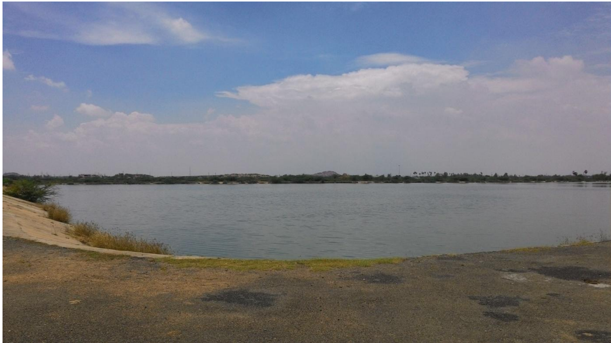
Figure 5: Waste Stabilisation Pond at Panjapur (Source: Bhitush/CSE, 2015)
