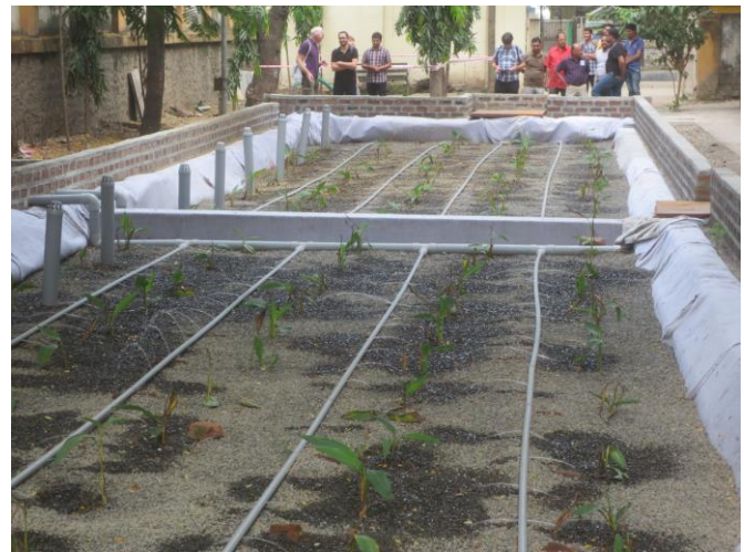
Fig. 8: VF basins for greywater treatment during start-up in COEP hostel (source: ESF; 2015)
