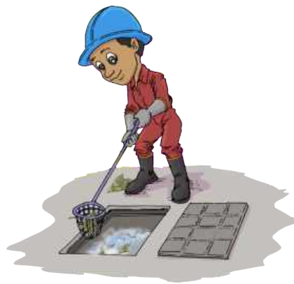
Removal of floating materials
