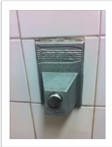
This hand dryer is less vulnerable to misuse or breakage because it is embedded in the wall.
