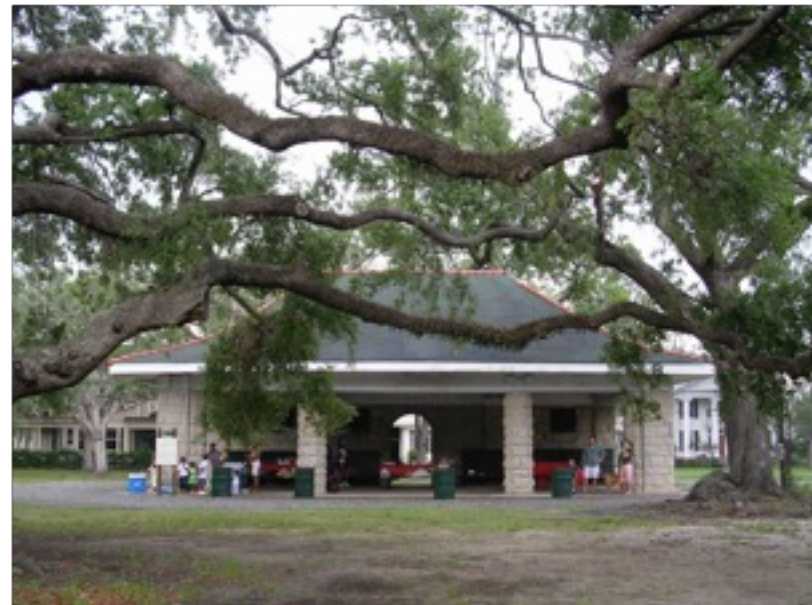
This restroom in a New Orleans park illustrates CPTED features: location near right of way, co-location with other public activities, and all around pedestrian circulation, including door through the middle to the toilet stalls.
