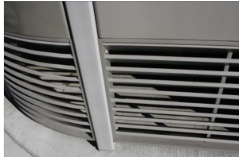
Angled slats at the bottom of the Portland Loo allow passers by and law enforcement to see if a user has fallen while not compromising privacy. Most toilet doors can be fitted with similar slats.
