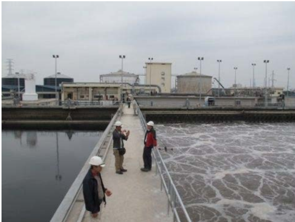
Picture of Yen So WWTP (Nguyen 2015)
