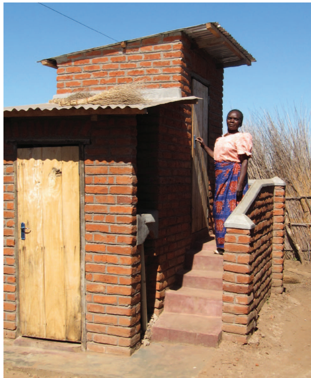
Figure 1. CCODE toilet, credit CCODE 2015
